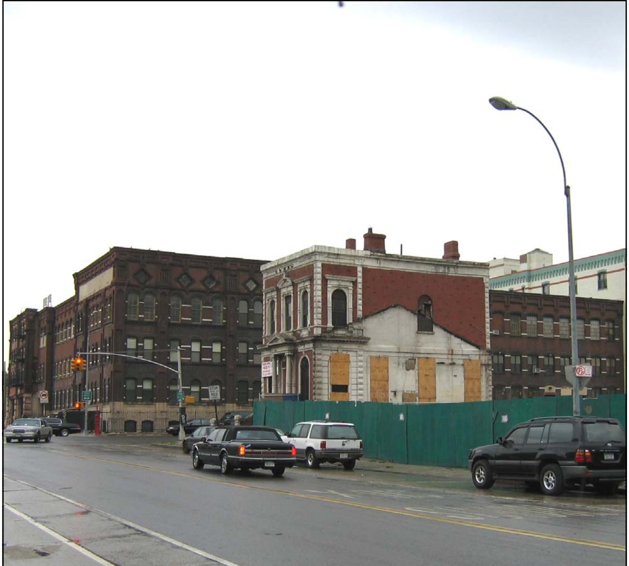
New York and Long Island Coignet Stone Company Building View from Third Street, west façade Photo: Matthew A. Postal
