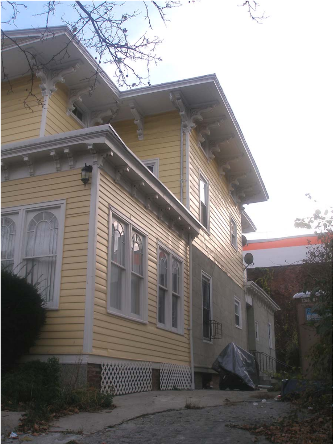
James W. and Lucy S. Elwell House, west façade.
