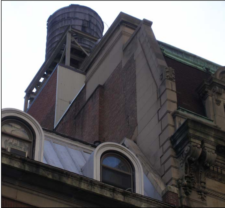
Henry Seligman Residence Exposed east façade party wall Photo: Amanda Davis
