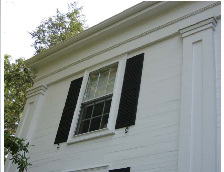
Window and trim detail Photo: Tara Harrison
