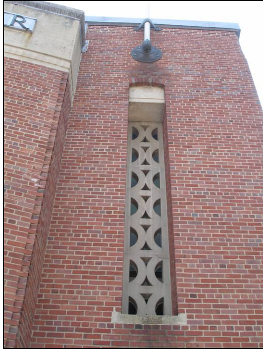
Detail: Cast stone
