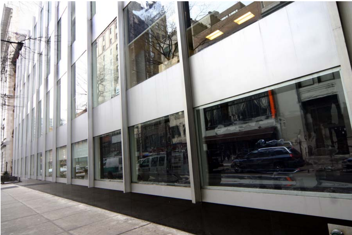
East 18 th Street facade, base, looking east
