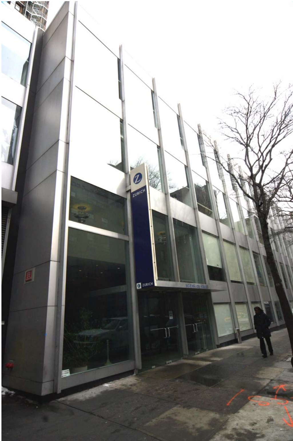
17 th Street entrance, looking east Photo by Carl Forster
