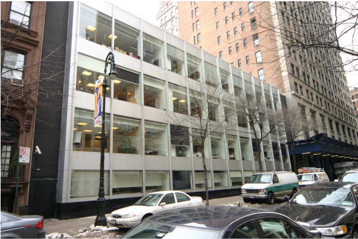
East 18 th Street facade, looking west Photos by Carl Forster
