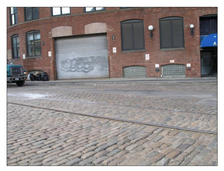
Figure 4 Rail tracks and Belgian block paving on Adams Street between Plymouth and Water Streets Photo: Jennifer L. Most
