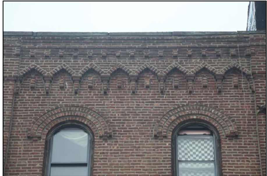
William Ulmer Brewery Engine and Machine House, Cornice Detail Photo: Christopher D, Brazee, 2009
