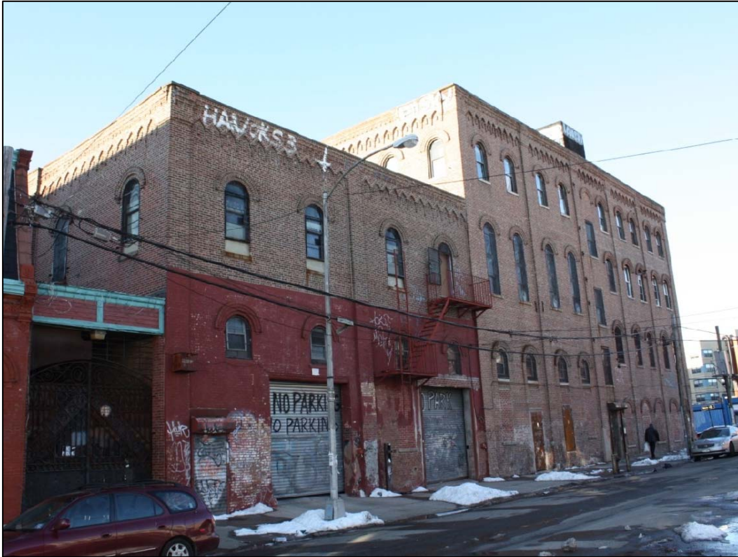
William Ulmer Brewery Engine and Machine House Photo: Tara Harrison, 2010
