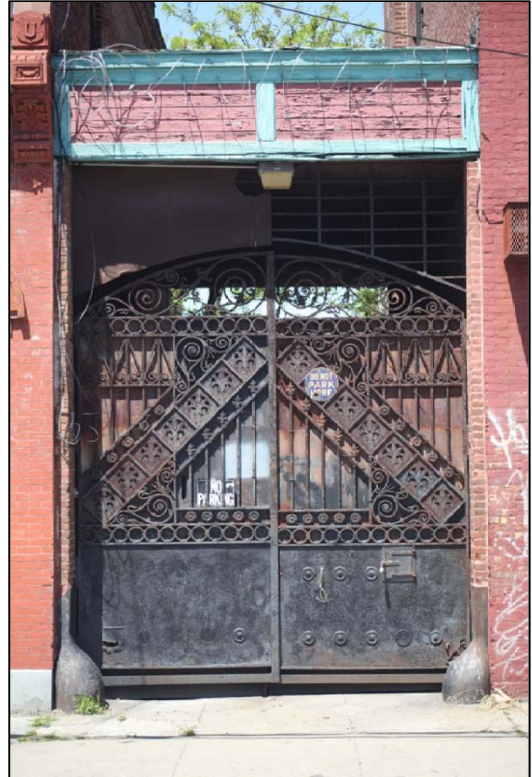
William Ulmer Brewery Office Building, Gate Photo: Christopher D. Brazee, 2010
