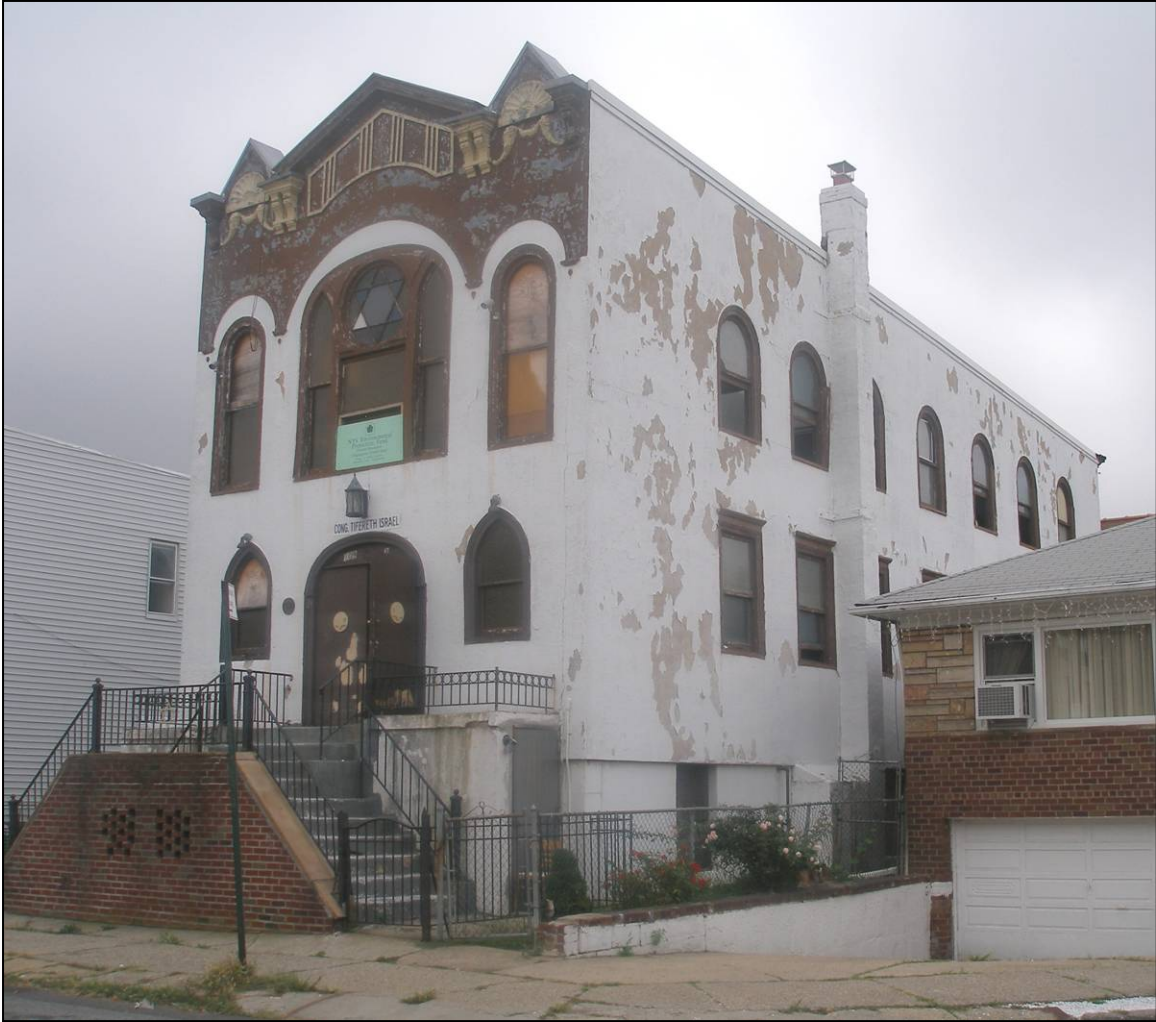
Congregation Tifereth Israel, main and west façades, view looking southeast Photo: Kathryn Horak
