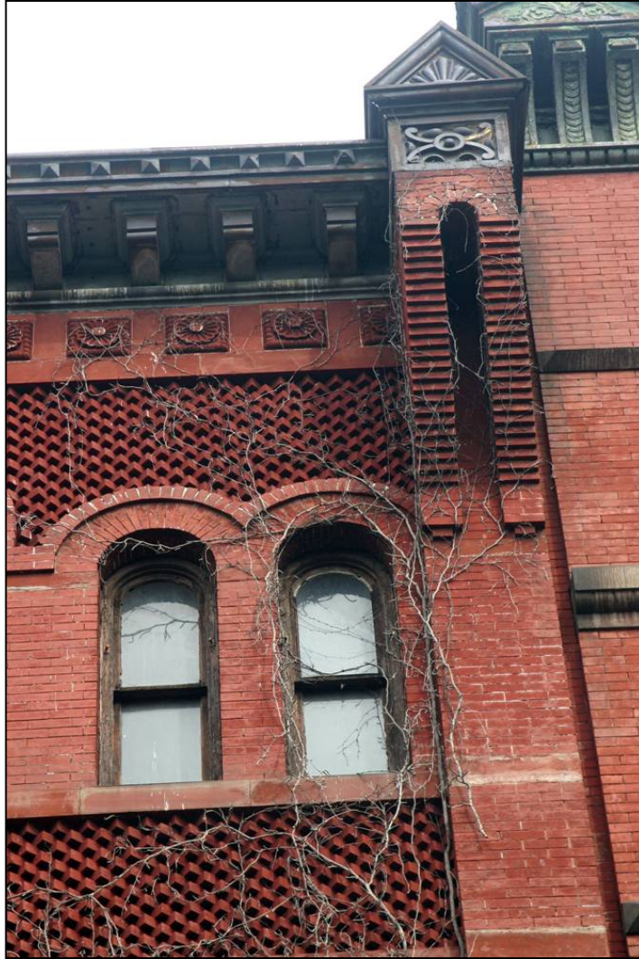
Fire Engine Company No. 53, 175 East 104 th Street Detail of Roof line Photo: Carl Forster
