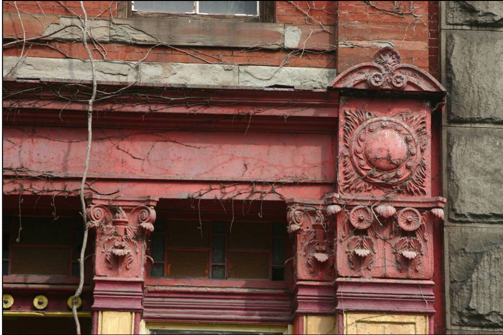
Fire Engine Company No. 53, 175 East 104 th Street Detail of base Photo: Carl Forster
