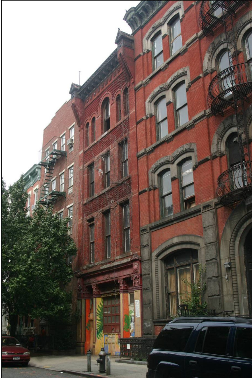
Fire Engine Company No. 53, 175 East 104 th Street Photo: Carl Forster
