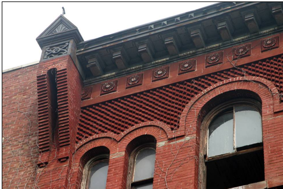
Fire Engine Company No. 53, 175 East 104 th Street Detail of roof line Photo: Carl Forster
