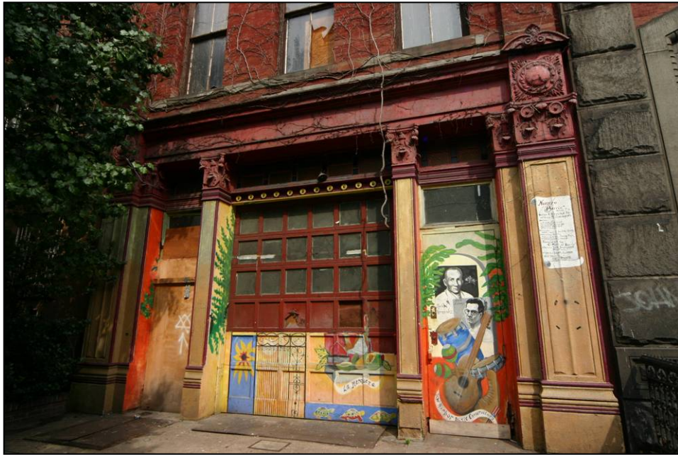
Fire Engine Company No. 53, 175 East 104 th Street Base of building Photo: Carl Forster
