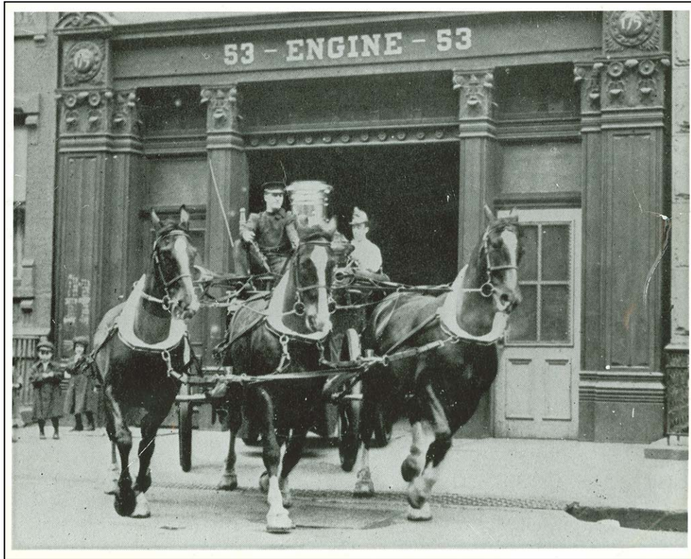
Fire Engine Company No. 53, 175 East 104 th Street Photo courtesy: Fire Department City of New York Mand Library and Learning Center
