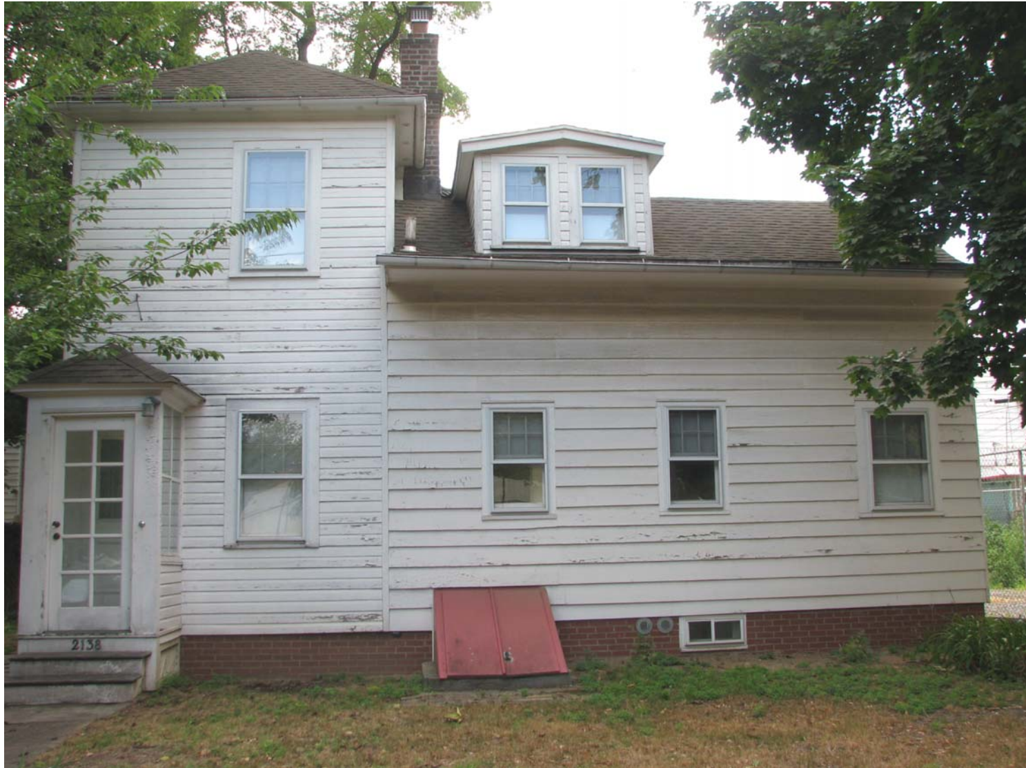
Hubbard House 2138 McDonald Avenue, Brooklyn Photo: Gale Harris, 2008
