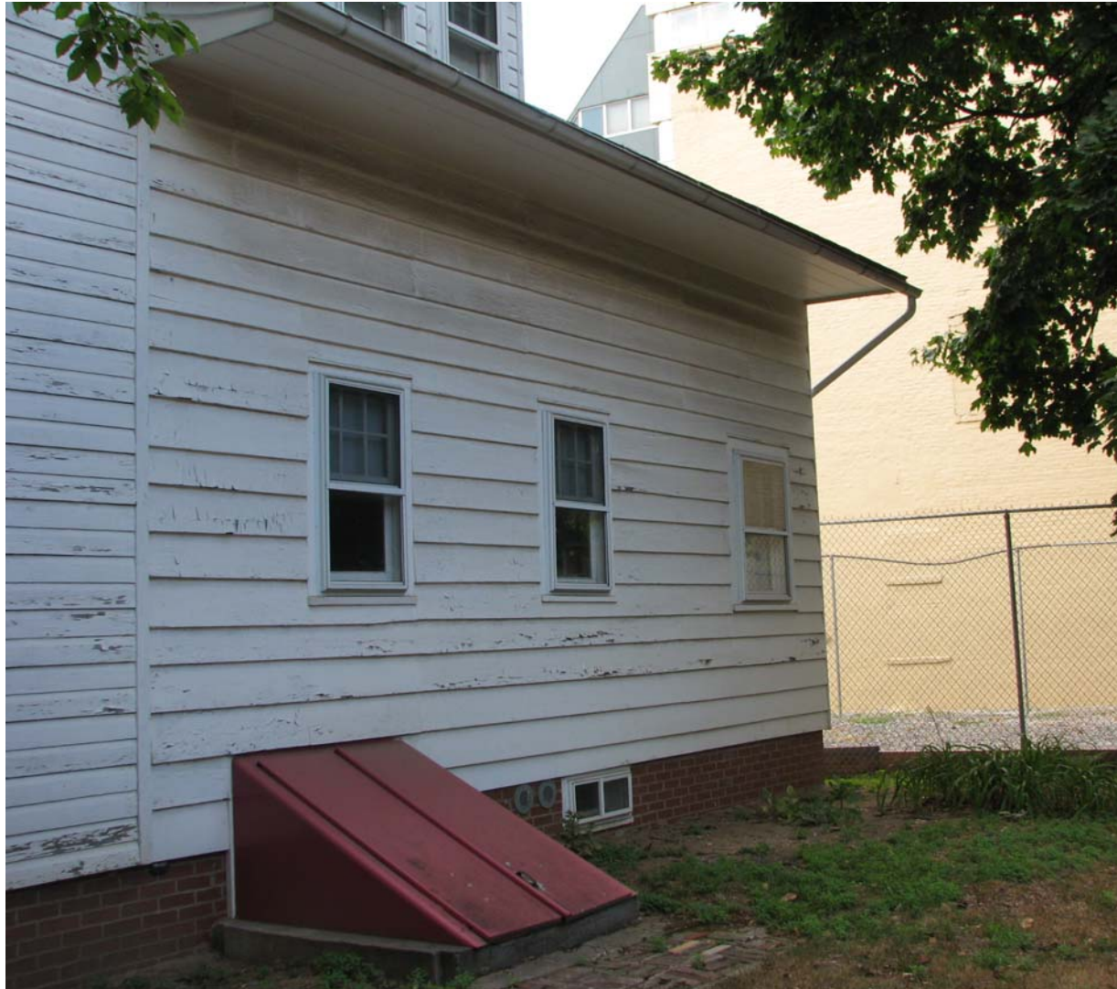
Hubbard House Spring eave, 1830s wing Photo: Gale Harris
