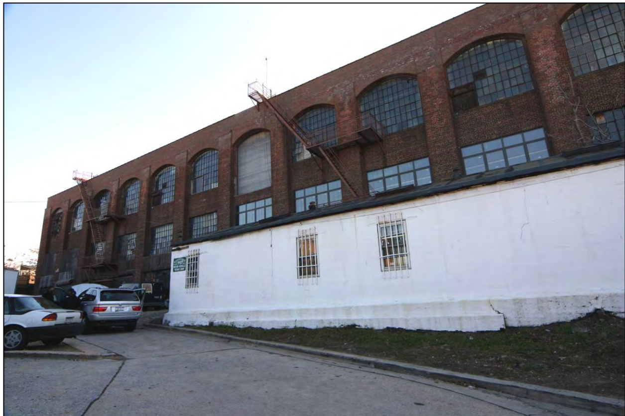
American Bank Note Company Printing Plant (Figure 18): Printing press wing, north facade (Photo: Carl Forster)
