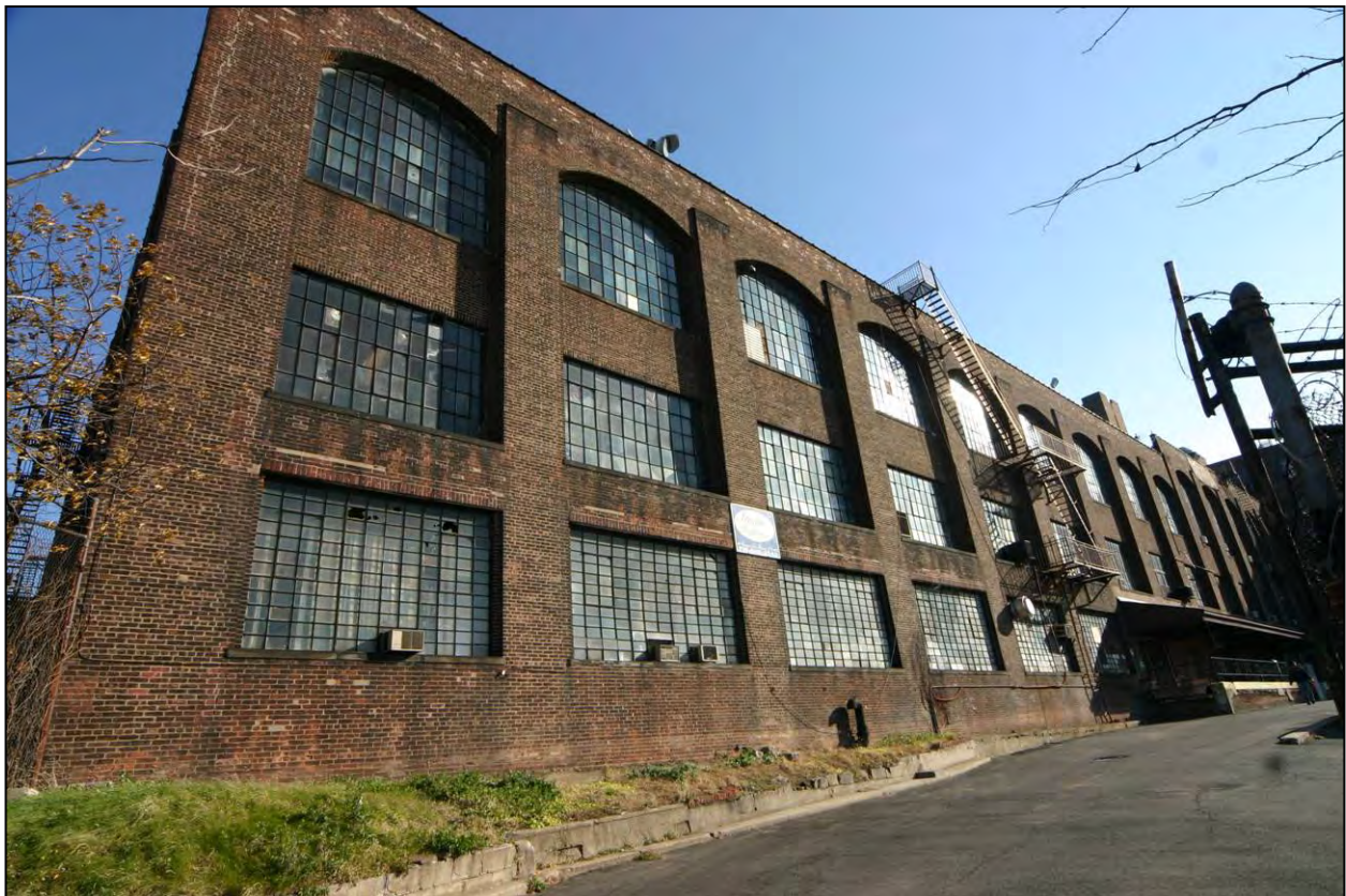
American Bank Note Company Printing Plant (Figure 13): Printing Press wing, west facade (Photo: Carl Forster)
