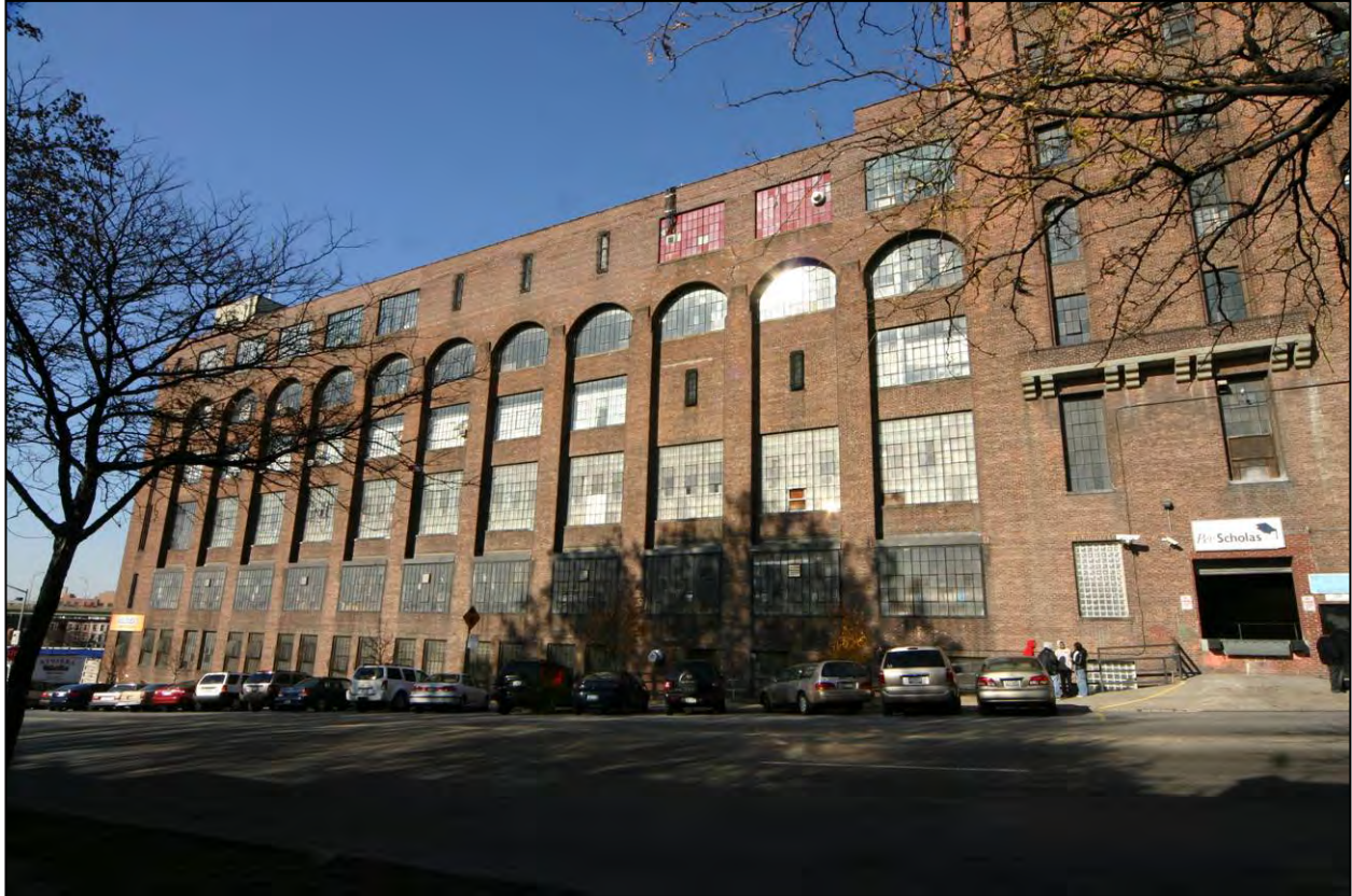
American Bank Note Company Printing Plant (Figure 6): Lafayette Avenue wing, south facade (Photo: Carl Forster)
