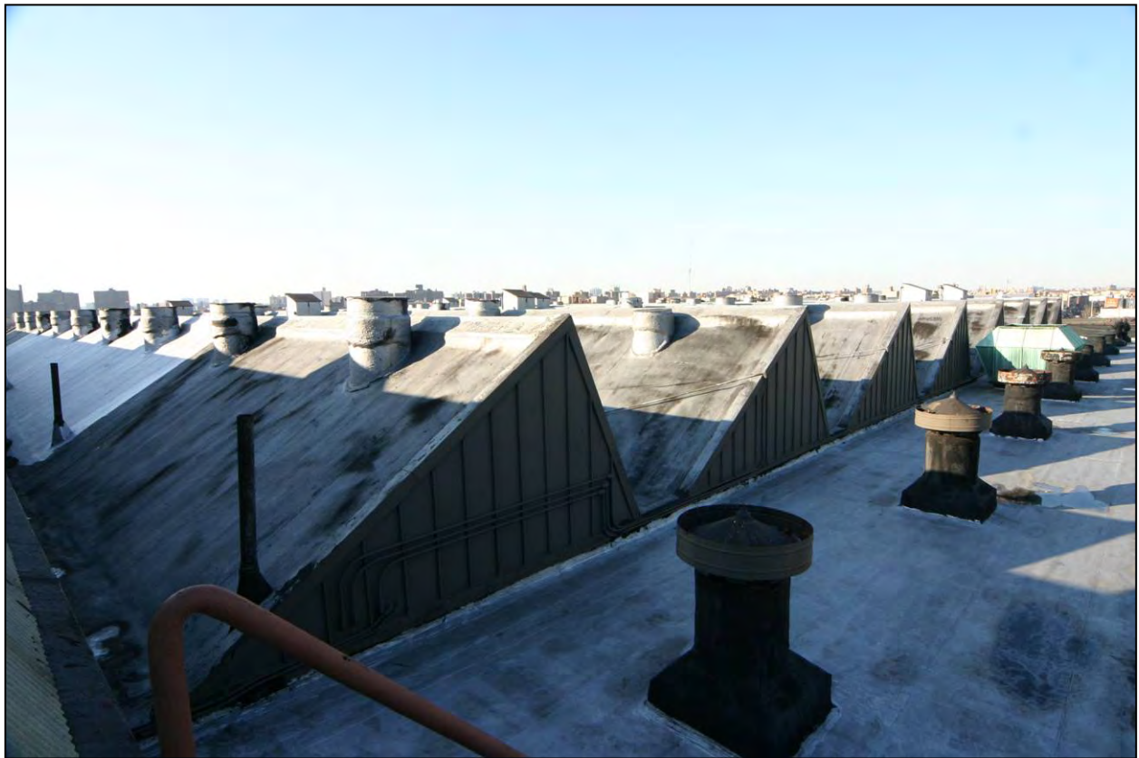
American Bank Note Company Printing Plant (Figure 26): Saw-tooth roof of Printing Press wing (Photo: Carl Forster)
