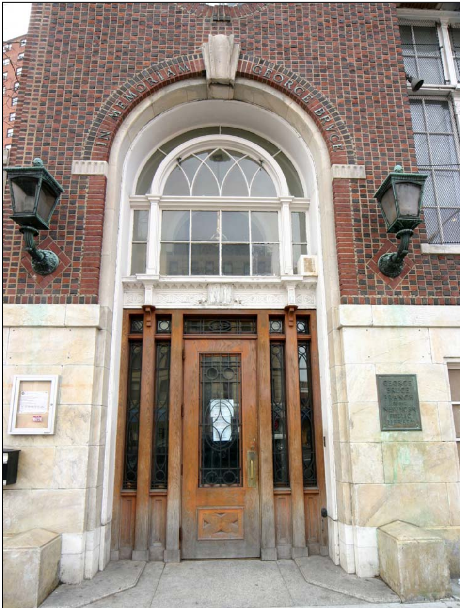
The New York Public Library, George Bruce Branch 518 West 125 th Street Main entrance detail Photo: Carl Forster
