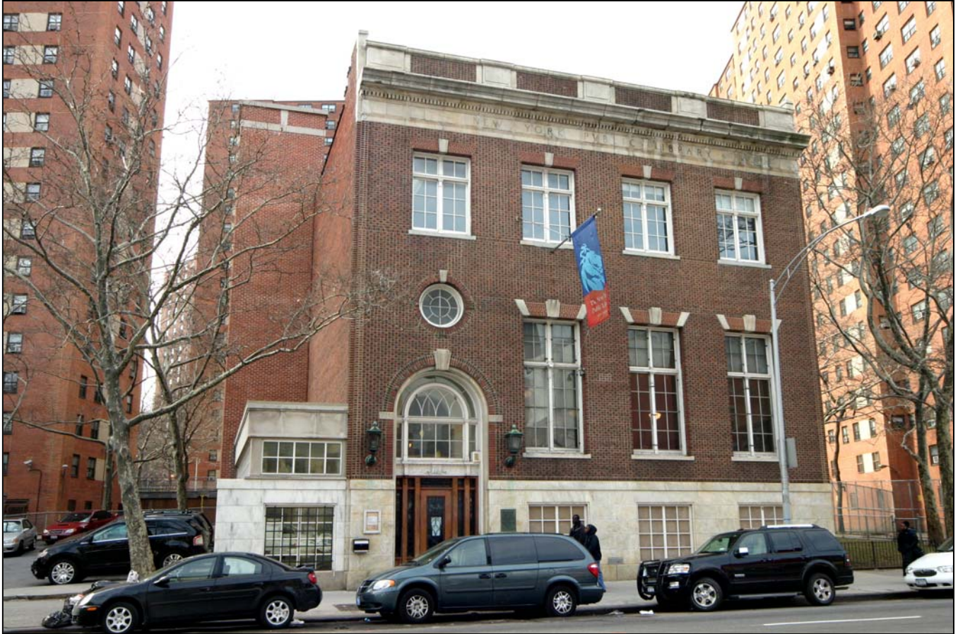
The New York Public Library, George Bruce Branch 518 West 125 th Street Main elevation (north) Photo: Carl Forster
