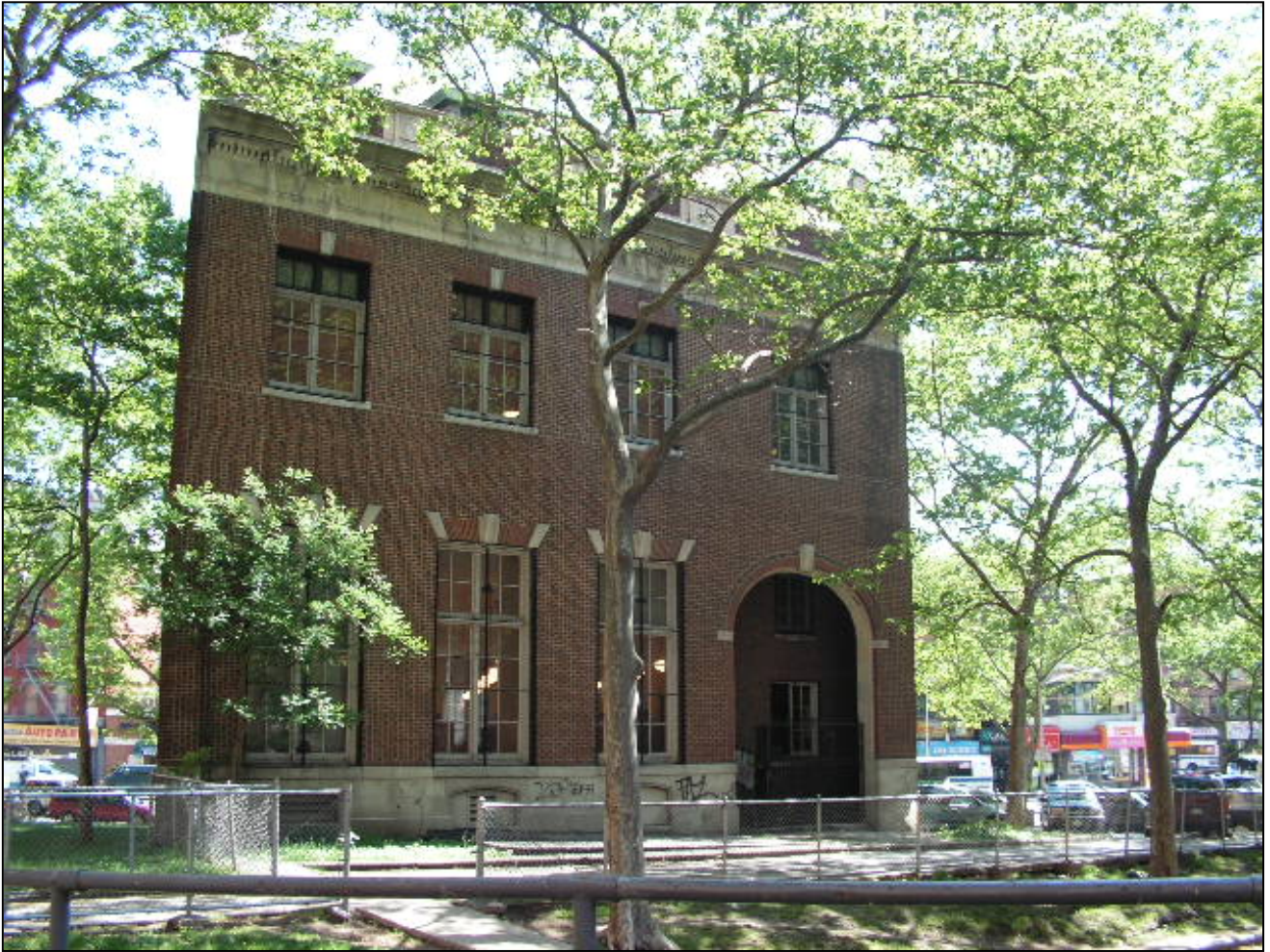
The New York Public Library, George Bruce Branch 518 West 125 th Street Rear elevation (south) Photo: Theresa C. Noonan
