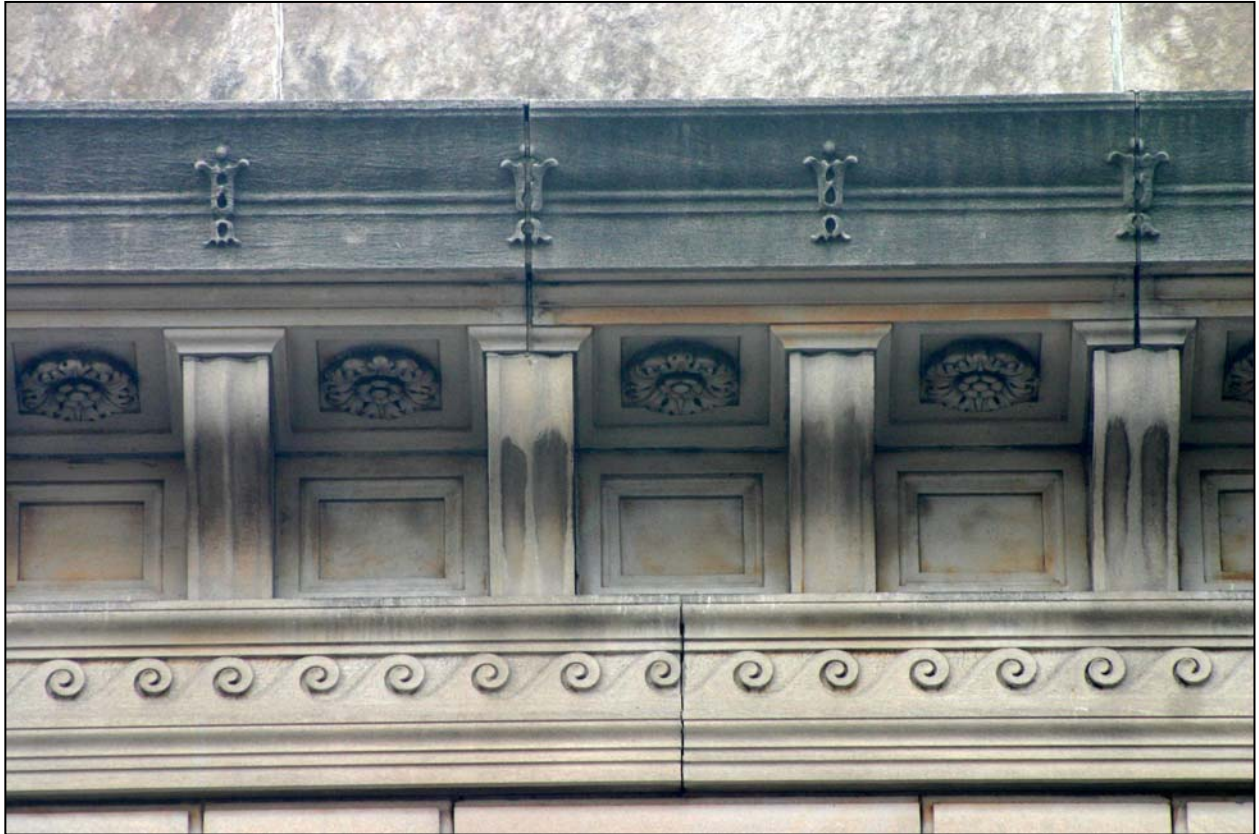
The New York Public Library, 125th Street Branch 224 East 125 th Street Cornice detail Photo: Carl Forster
