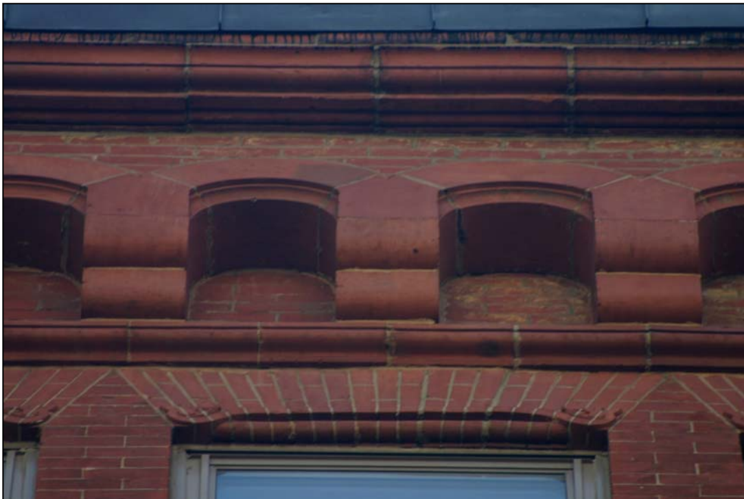
F.W. Devoe & Co. Factory Detail of terra-cotta arches in cornice Photo: Christopher D. Brazee (2008)
