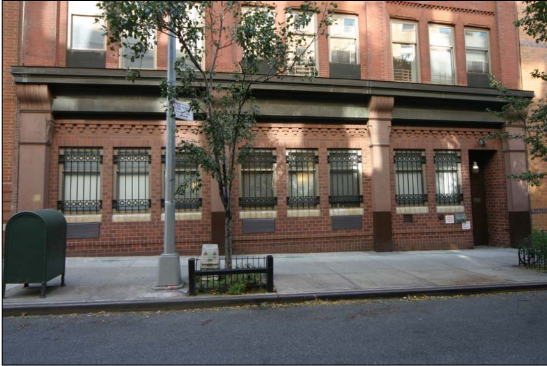
F.W. Devoe & Co. Factory Detail of ground floor Photo: Christopher D. Brazee (2008)
