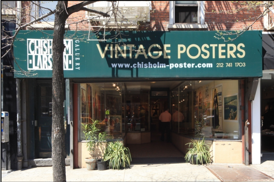
145 Eighth Avenue Storefront Detail
