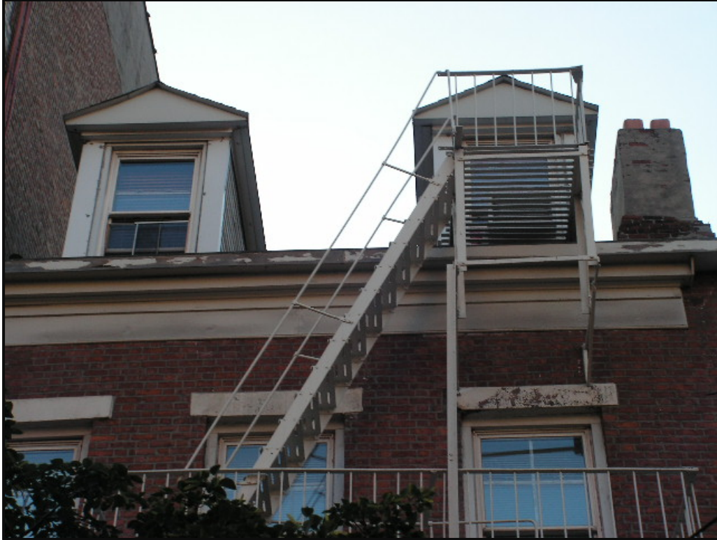
145 Eighth Avenue Roof Detail Photo: Theresa C. Noonan, 2009
