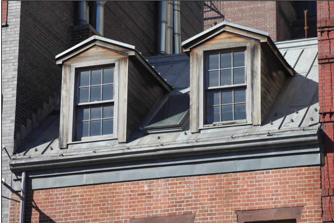
143 Allen Street House Detail of attic story with pitched roof and dormers Photo: Christopher D. Brazee (2010)
