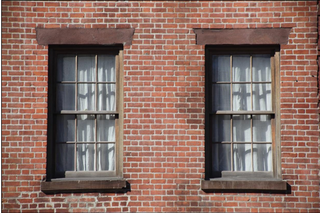
143 Allen Street House Detail of second story windows and Flemish bond brickwork Photo: Christopher D. Brazee (2010)
