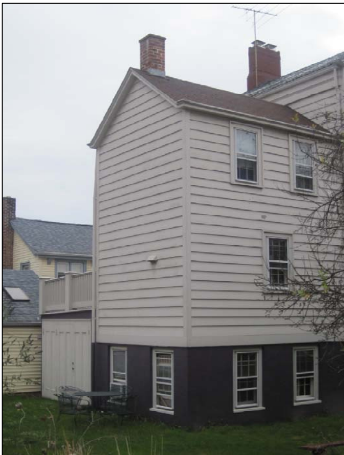
Mary and David Burgher House West and north facades of addition and rear deck Photo: Tara Harrison, 2009
