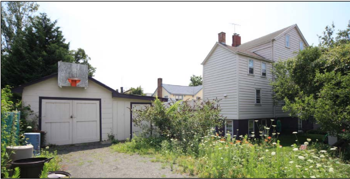
Mary and David Burgher House Rear addition and garage Photo: Christopher D. Brazee, 2009
