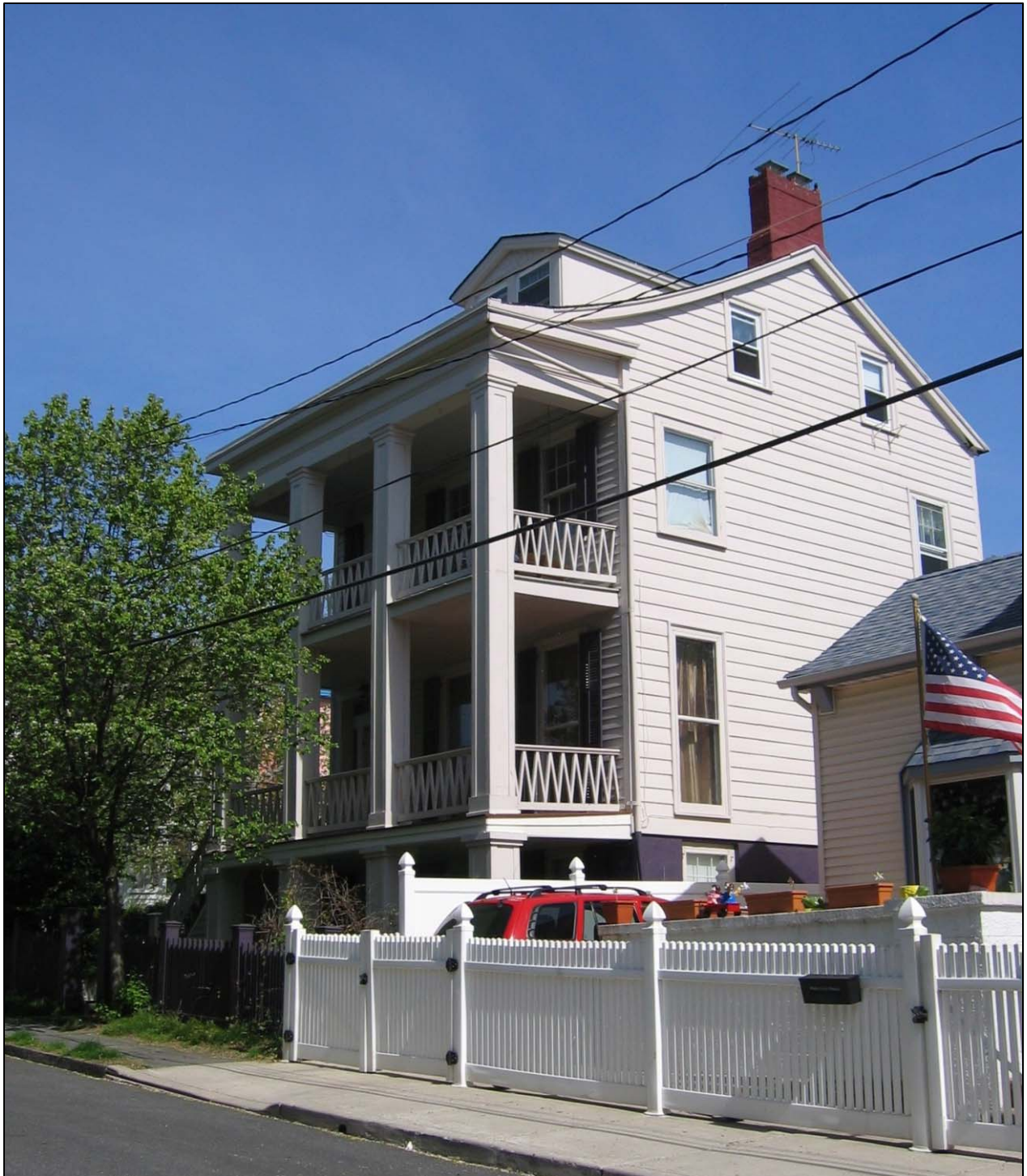
Mary and David Burgher House South and east facades Photo: Tara Harrison, 2009
