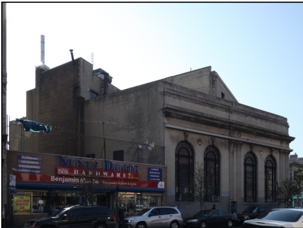
Dollar Savings Bank, (northern facade) Photo: Christopher D. Brazee, 2009
