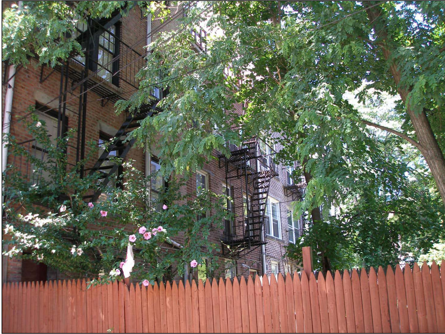
415-411 Westervelt Avenue, Rear Facades Photo: Tara Harrison, 2009
