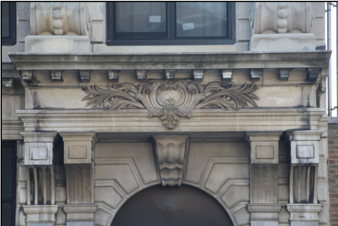
Haffen Building Third Avenue Facade (Details) Photos: Christopher D. Brazee, 2009
