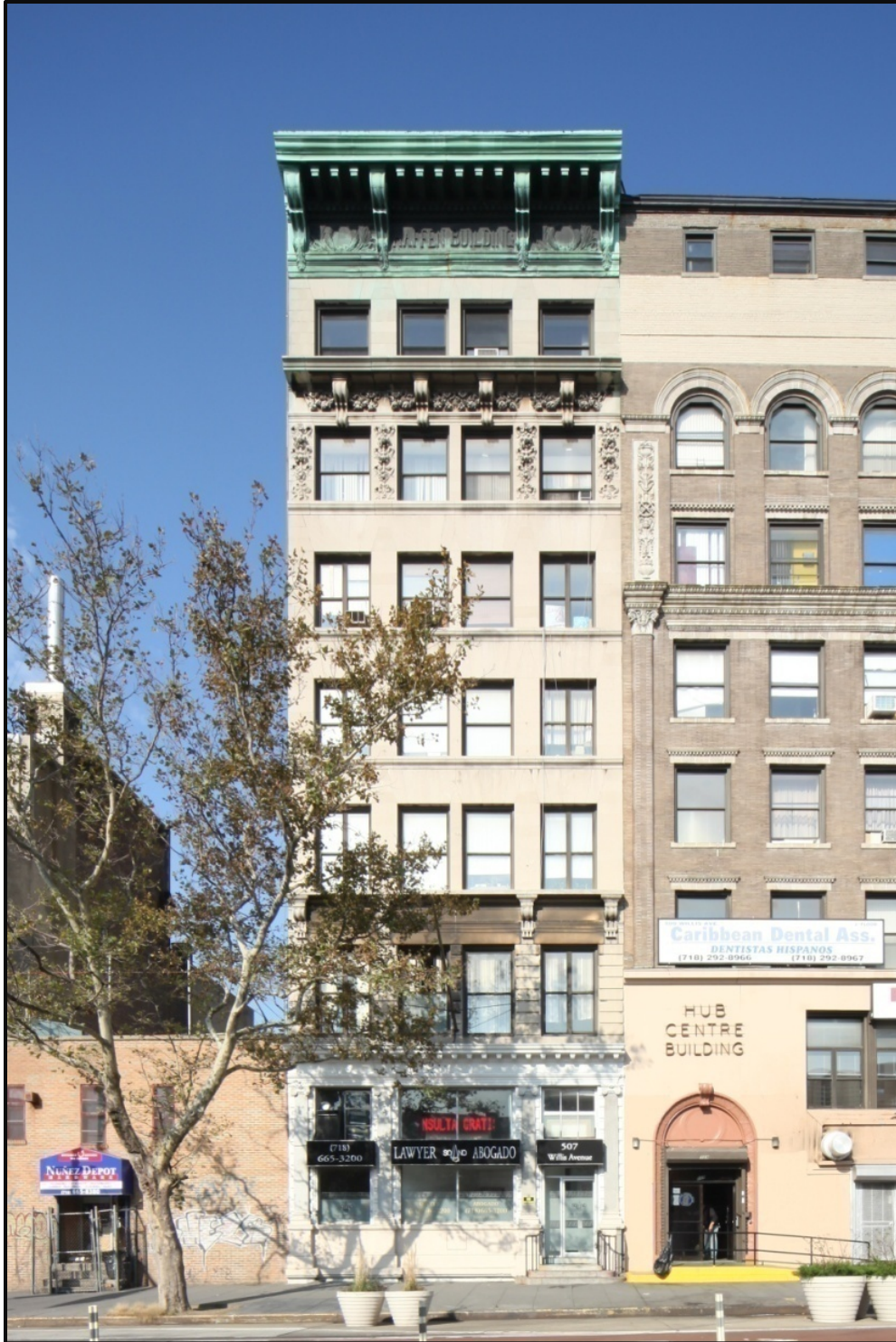
Haffen Building Willis Avenue Facade Photo: Christopher D. Brazee, 2009
