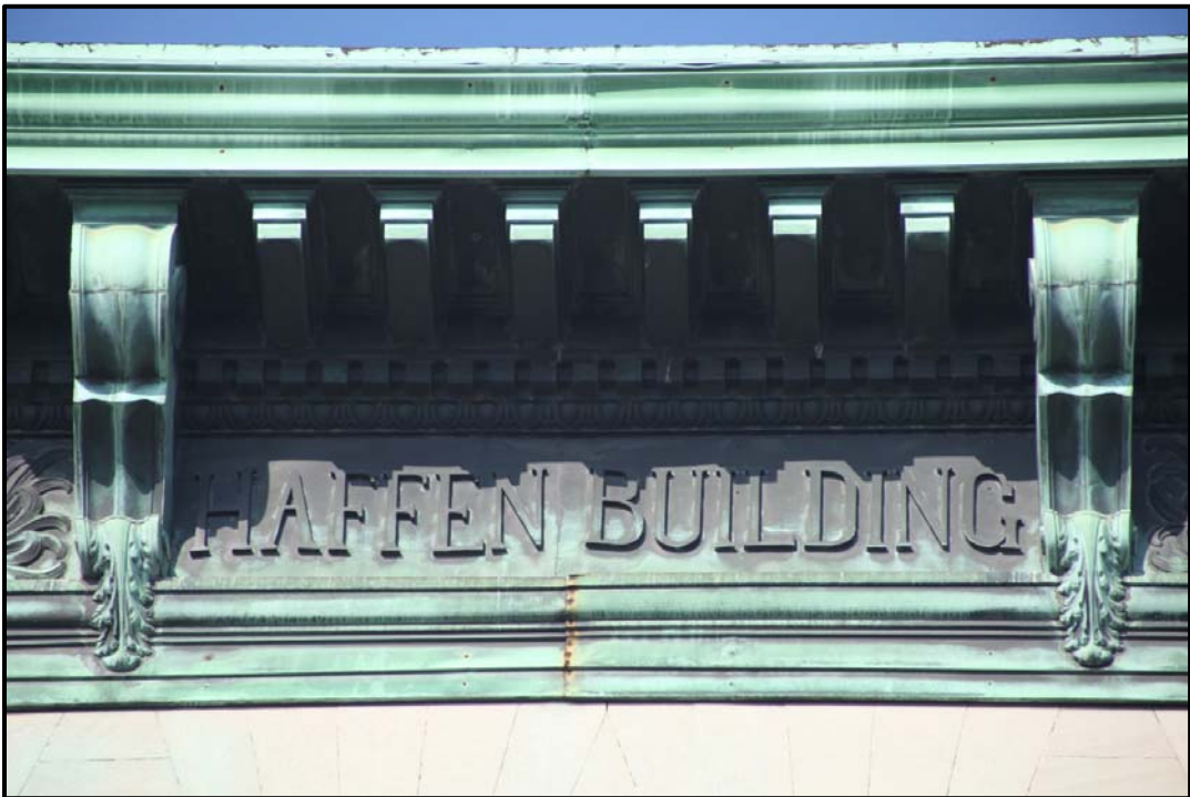
Haffen Building Willis Avenue Facade (Details) Photos: Christopher D. Brazee, 2009
