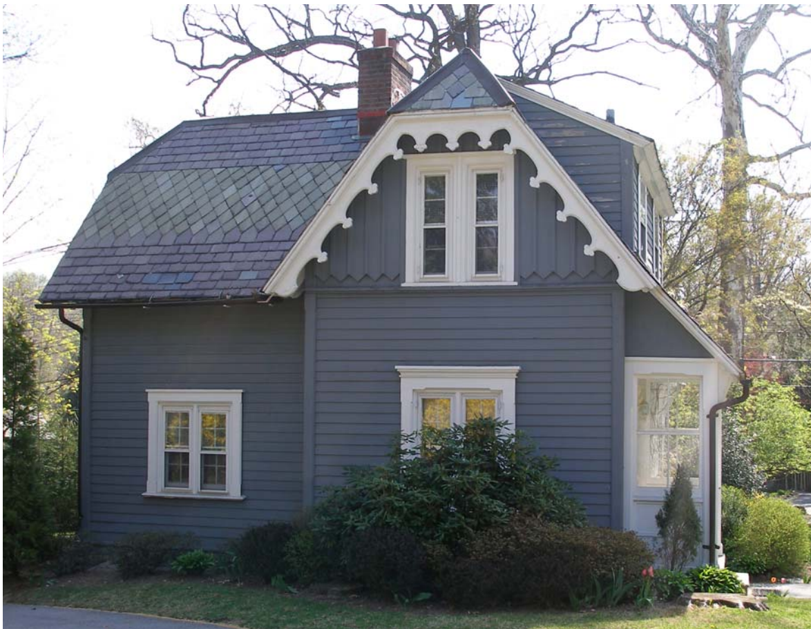
Greyston Gatehouse , from the southwest (upper) and west façade (lower)
