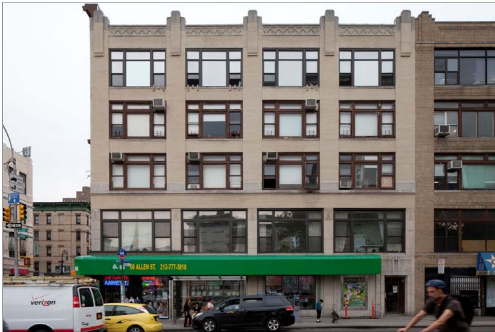
Edward Ridley & Sons Department Store Buildings 315-317 Grand Street, southeast corner of Allen Street (top) 315-317 Grand Street, view from Allen Street (bottom) Photo: Christopher D. Brazee, 2012
