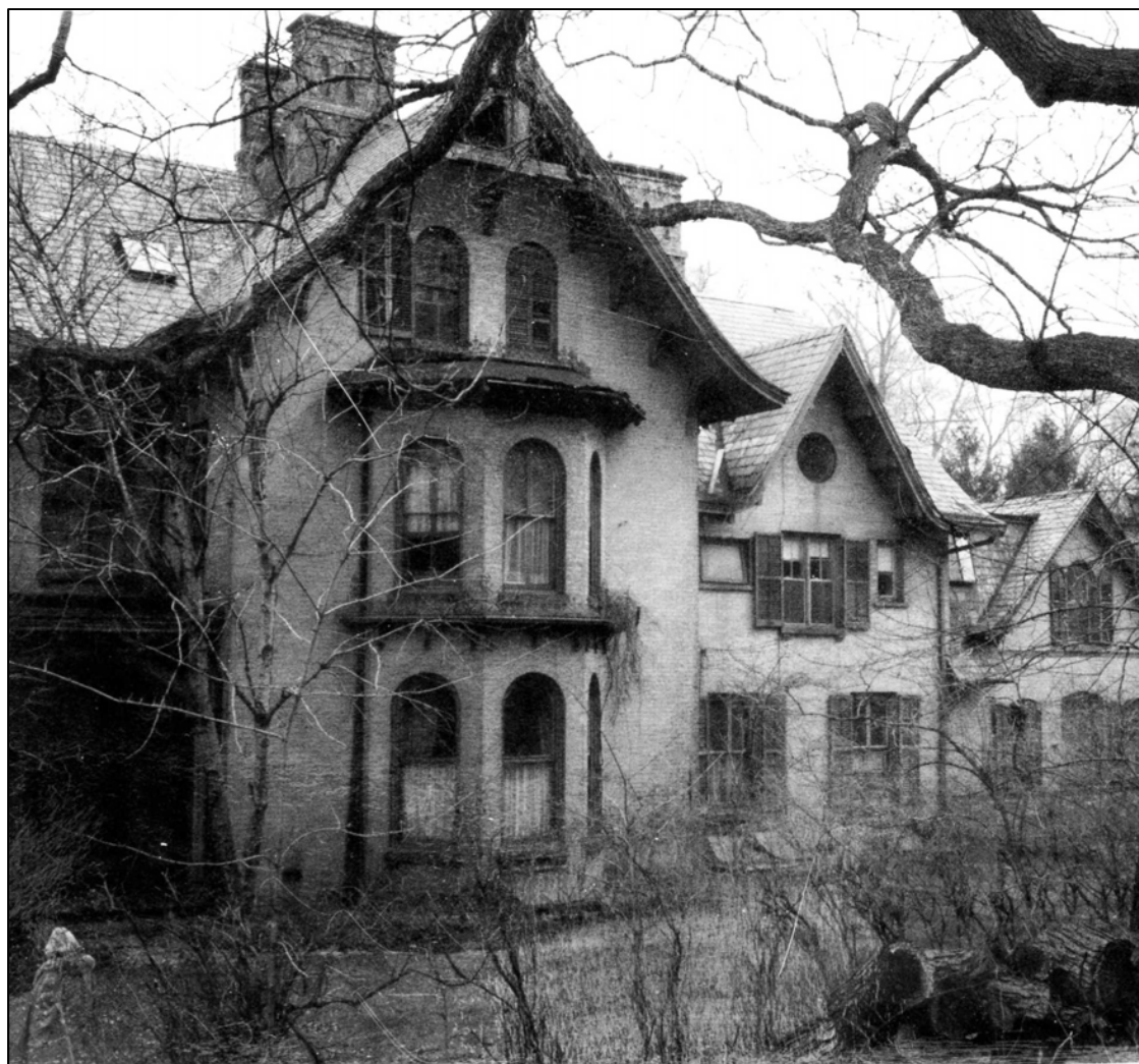
Alderbrook House South Facade, 1970 Photo: LPC
