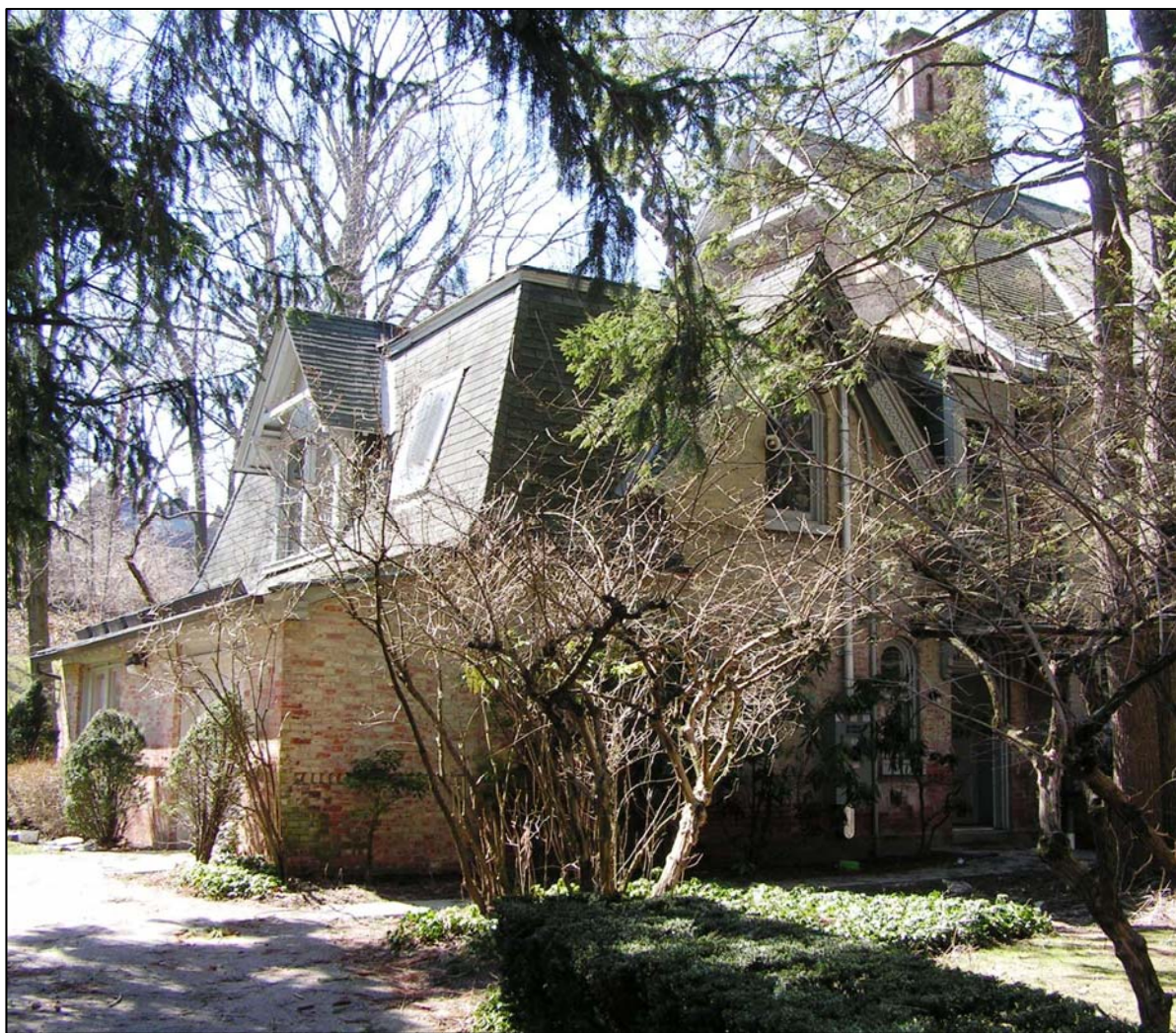
Alderbrook House East and North Facades of Eastern Wing Photo: Michael D. Caratzas, 2010
