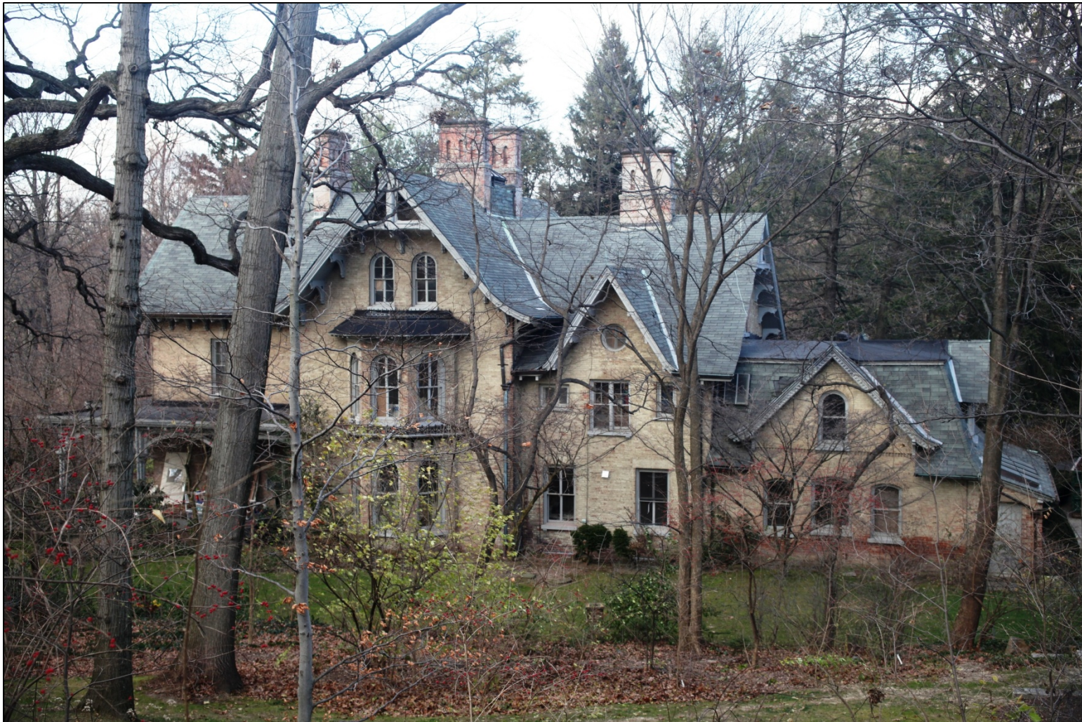
Alderbrook House 4715 Independence Avenue, the Bronx Block 5926, Lot 76 South Facade Photo: Michael D. Caratzas, 2009
