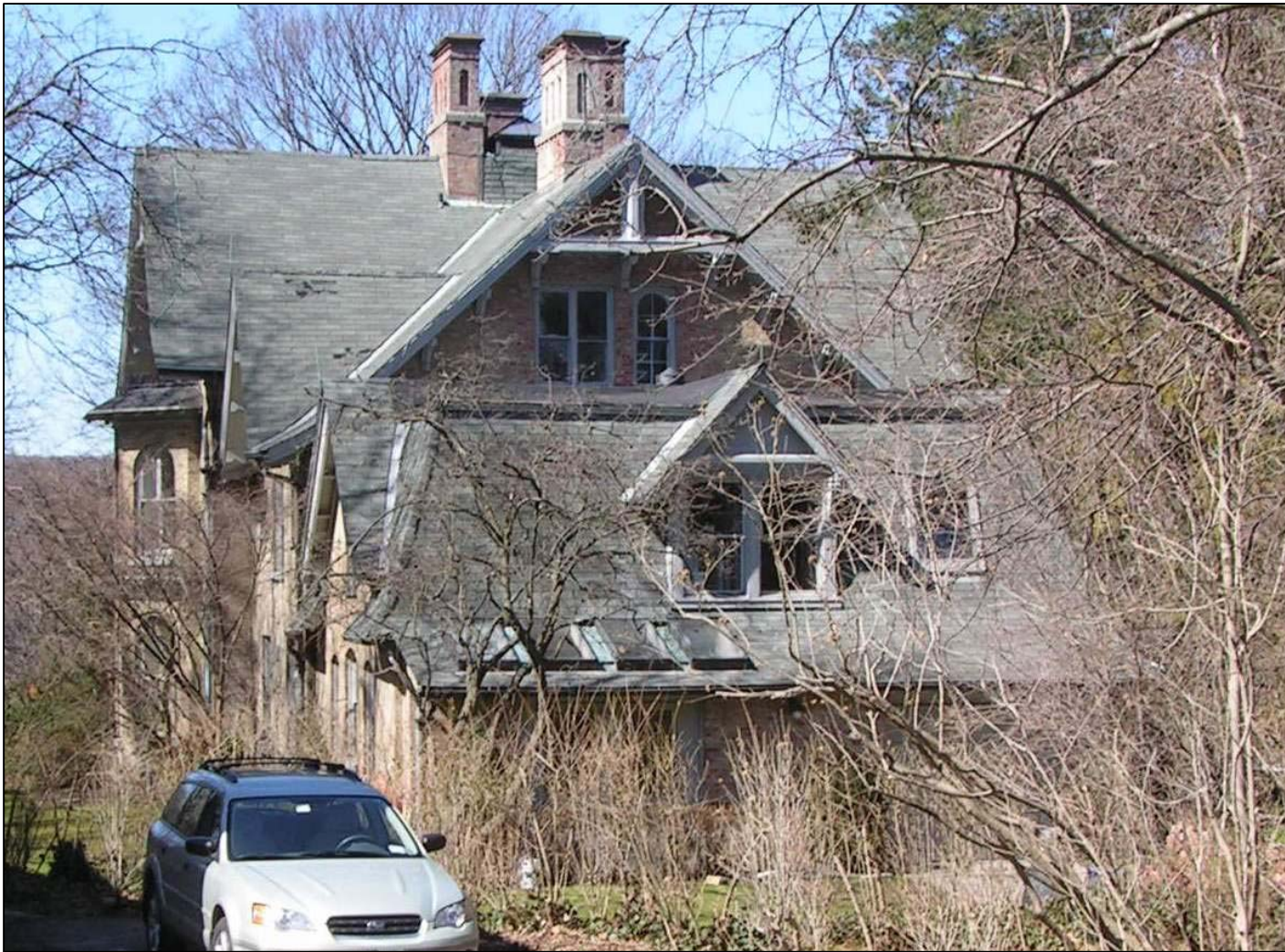
Alderbrook House East Facade of House and East Facade of Eastern Wing Photo: Michael D. Caratzas, 2010
