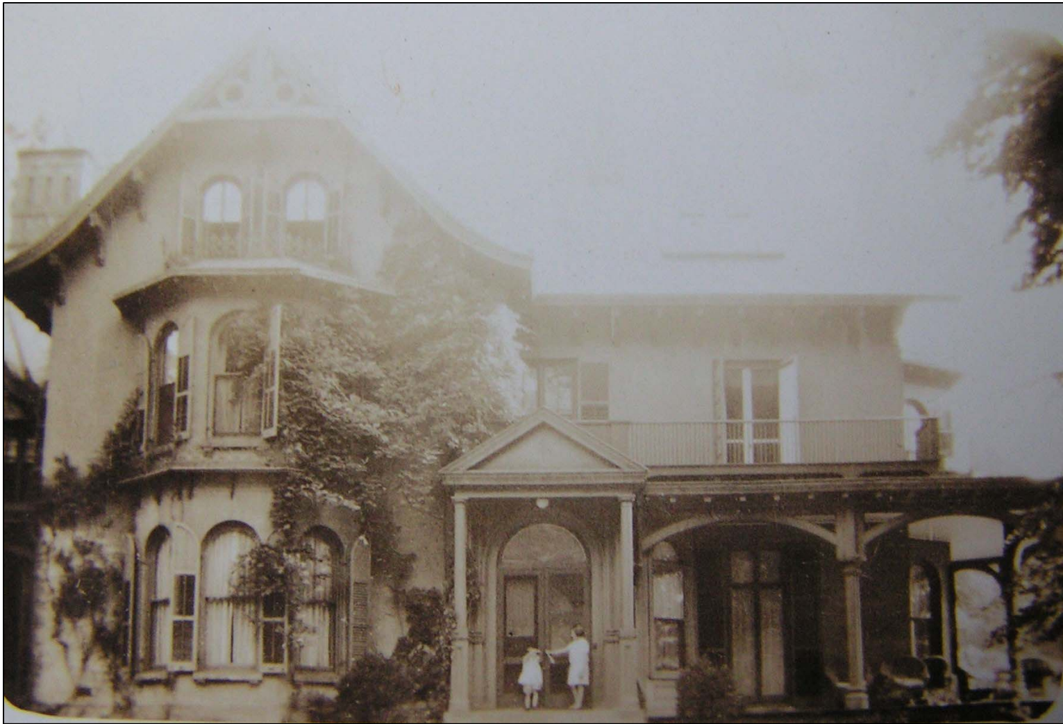
Alderbrook House North Facade, c.1927 Photo Courtesy of Cynthia Nadelman
