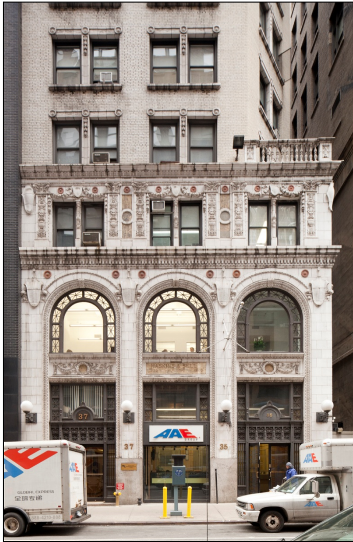
Haskins & Sells Building South (West 39 th Street) Facade: First through Fifth Stories Photo: Christopher D. Brazee, 2011 (Figure 4)
