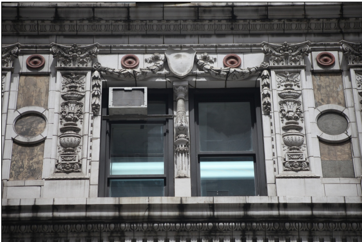
Haskins & Sells Building South (West 39 th Street) Facade: Fourth-Story Detail Photo: Christopher D. Brazee, 2010 (Figure 7)
