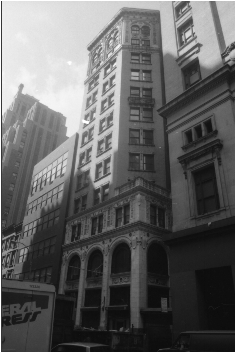
Haskins & Sells Building Looking Northwest from West 39 th Street Photo: LPC, Urban Cultural Resources Survey, 1985 (Figure 3)
