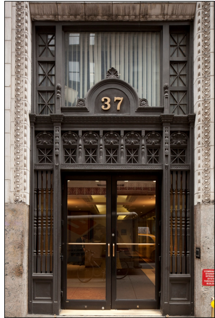
Haskins & Sells Building South (West 39 th Street) Facade: Door Detail Photo: Christopher D. Brazee, 2011 (Figure 5)
