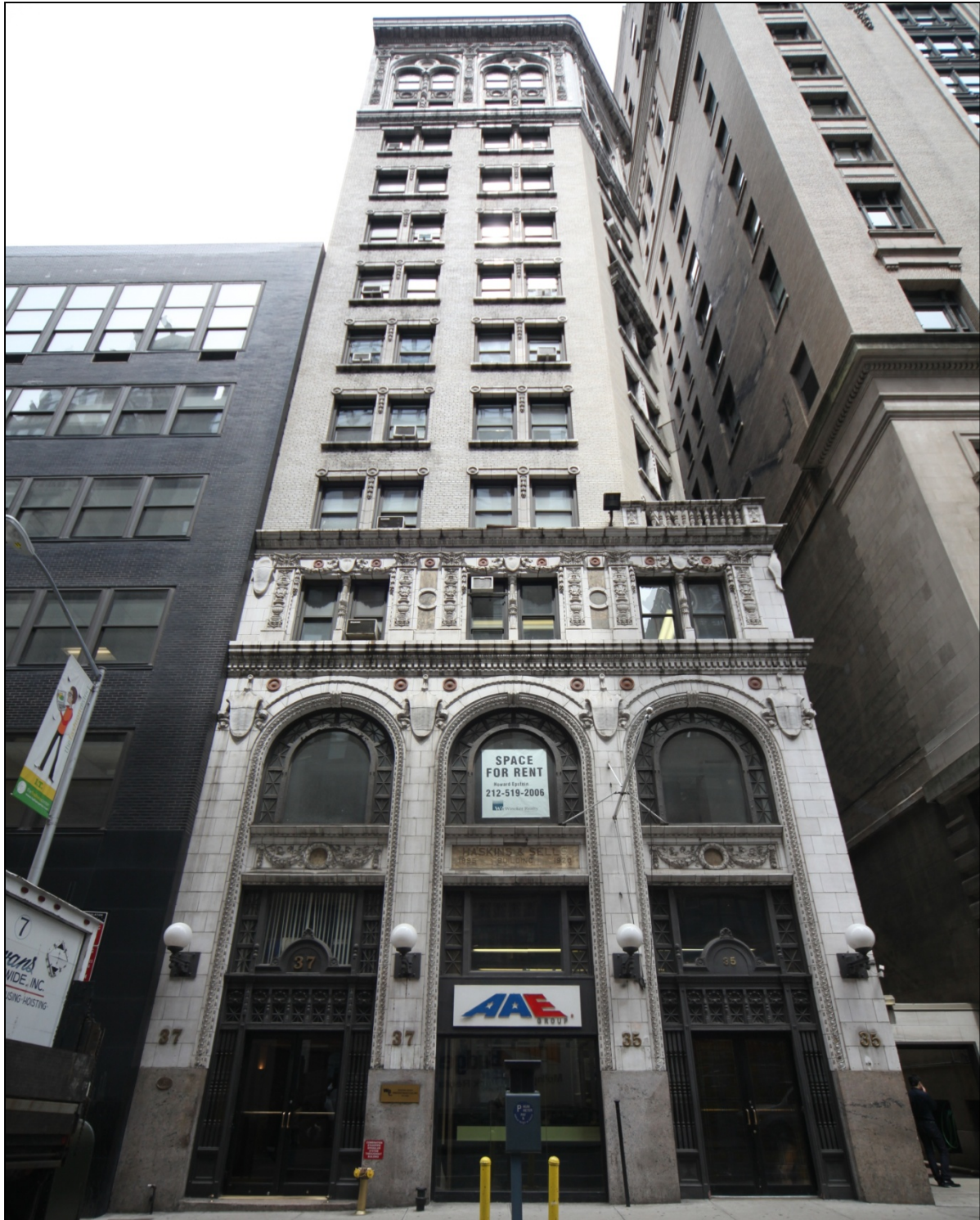
Haskins & Sells Building 35 West 39 th Street (aka 35-37 West 39 th Street) Borough of Manhattan, Tax Map Block 841, Lot 18 South (West 39 th Street) Facade Photo: Christopher D. Brazee, 2010 (Figure 1)
