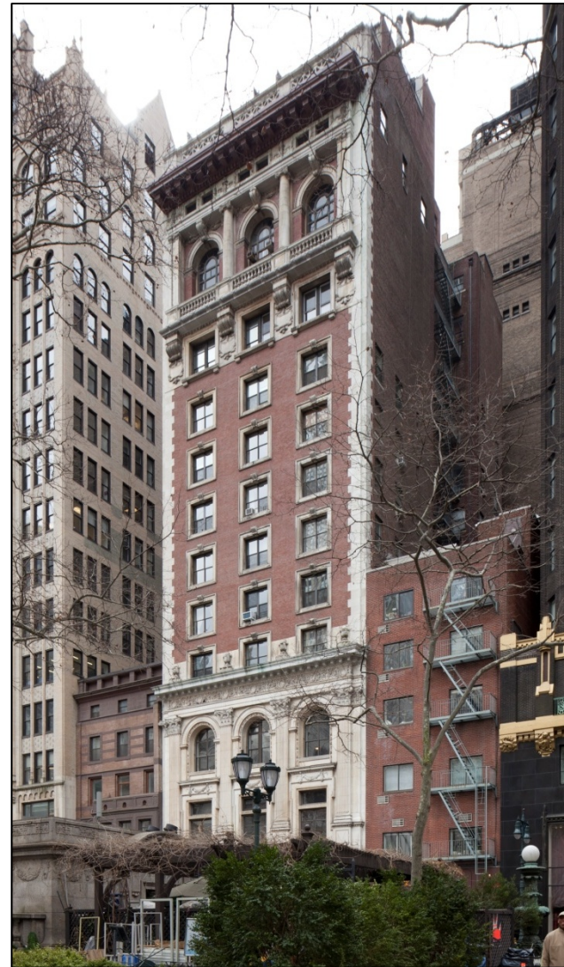
Engineers' Club Building North and West Facades Photo: Christopher D. Brazee, 2011
