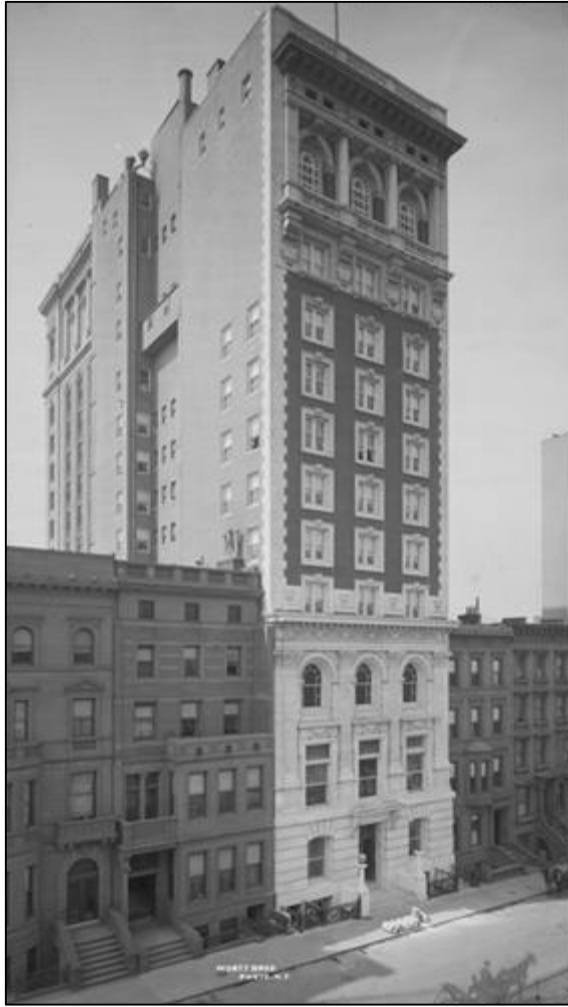
Engineers' Club Building, c. 1905 North and East Facades with Streetscape Courtesy of: Museum of the City of New York
