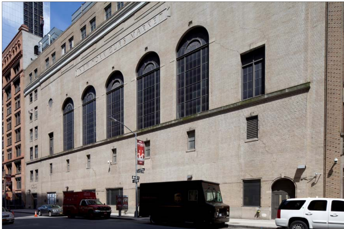
New York Curb Exchange Greenwich Street facade, view south and north Photos: Christopher D. Brazee, 2012
