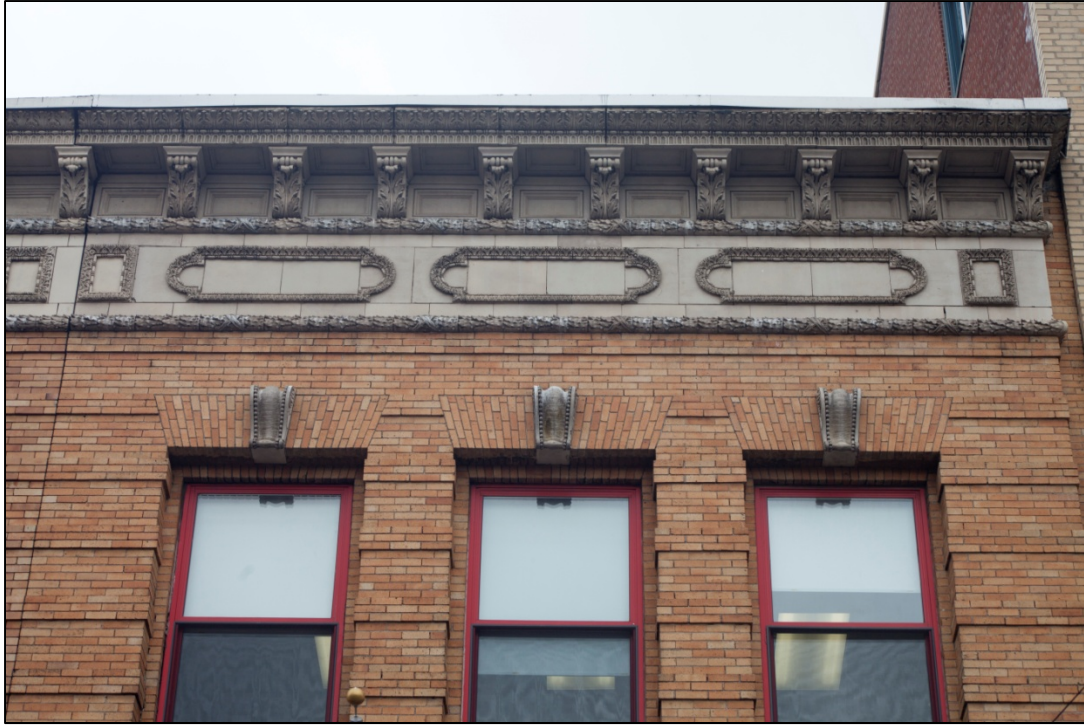
Firehouse, Engine Company 46 (now Engine Company 46/ Hook & Ladder Company 17) Details of terra cotta and brick work Photos: Christopher D. Brazee, 2013
