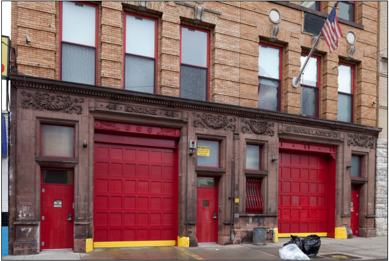
Firehouse, Engine Company 46 (now Engine Company 46/ Hook & Ladder Company 17) Ground story details Photo: Christopher D. Brazee, 2013
