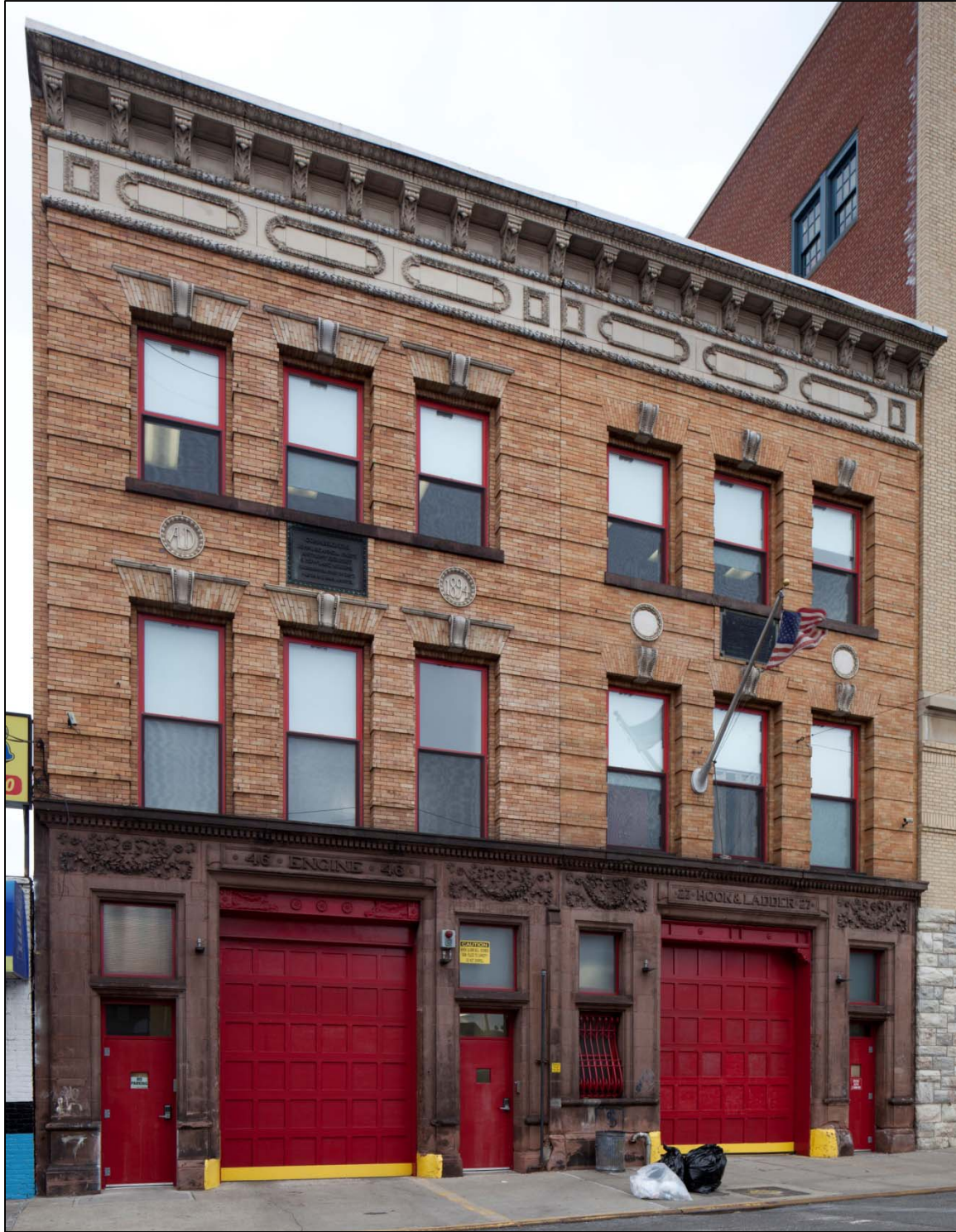
Firehouse, Engine Company 46 (now Engine Company 46/ Hook & Ladder Company 17) 451-453 East 176 th Street, Borough of the Bronx Block 2902/ Lot 40 Photo: Christopher D. Brazee, 2013
