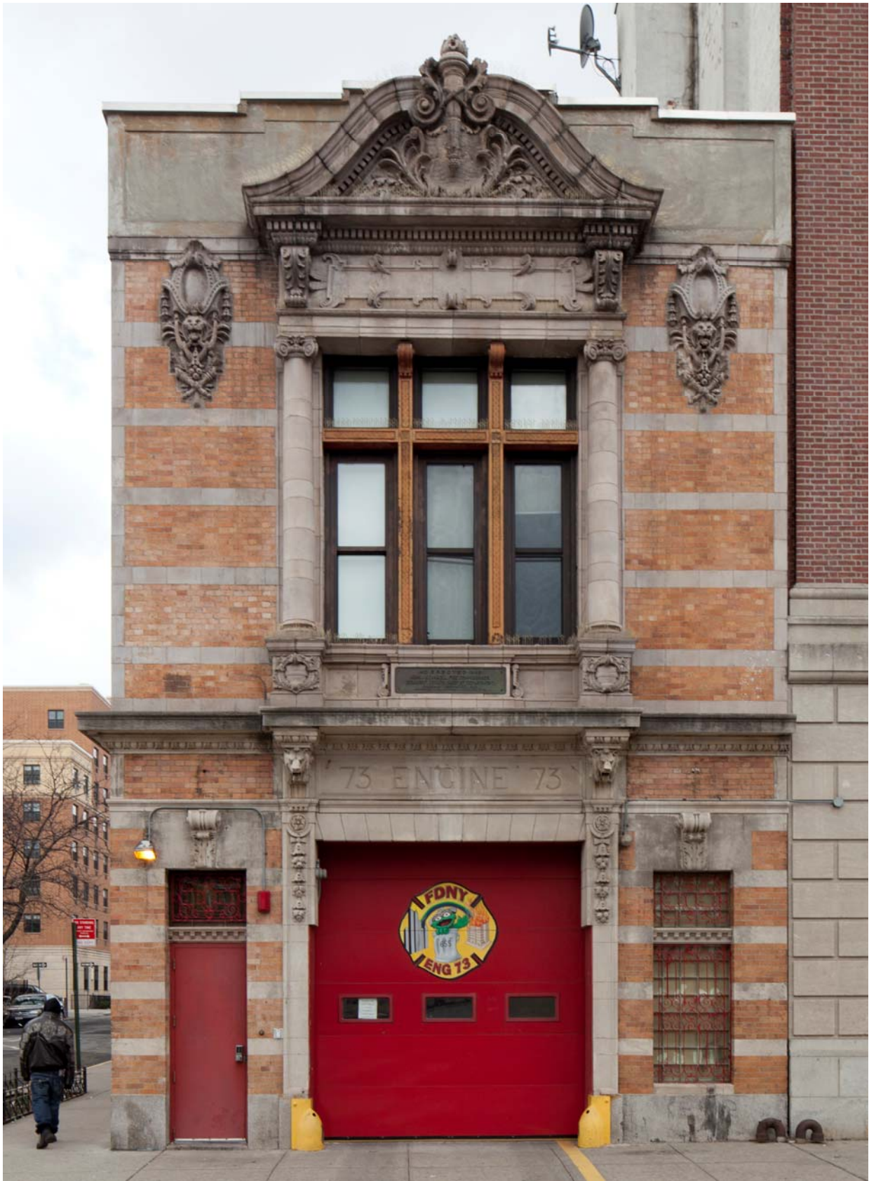
Firehouse, Engine Company 73
