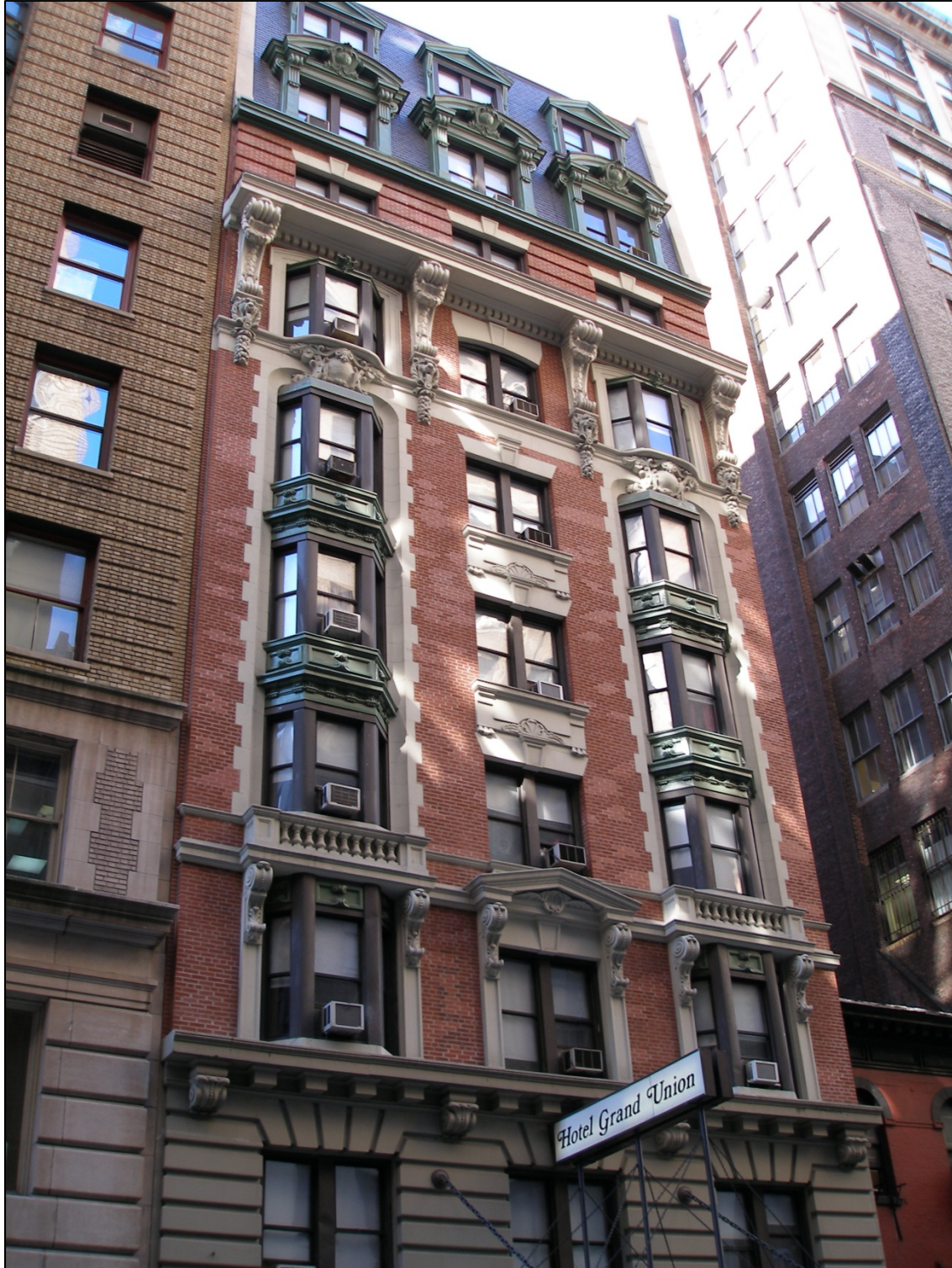
ST. LOUIS HOTEL (now HOTEL GRAND UNION) 34 East 32 nd Street (aka 34-36 East 32 nd Street), Manhattan Borough of Manhattan Tax Map Block 861, Lot 52 Photo: Theresa C. Noonan, 2006
