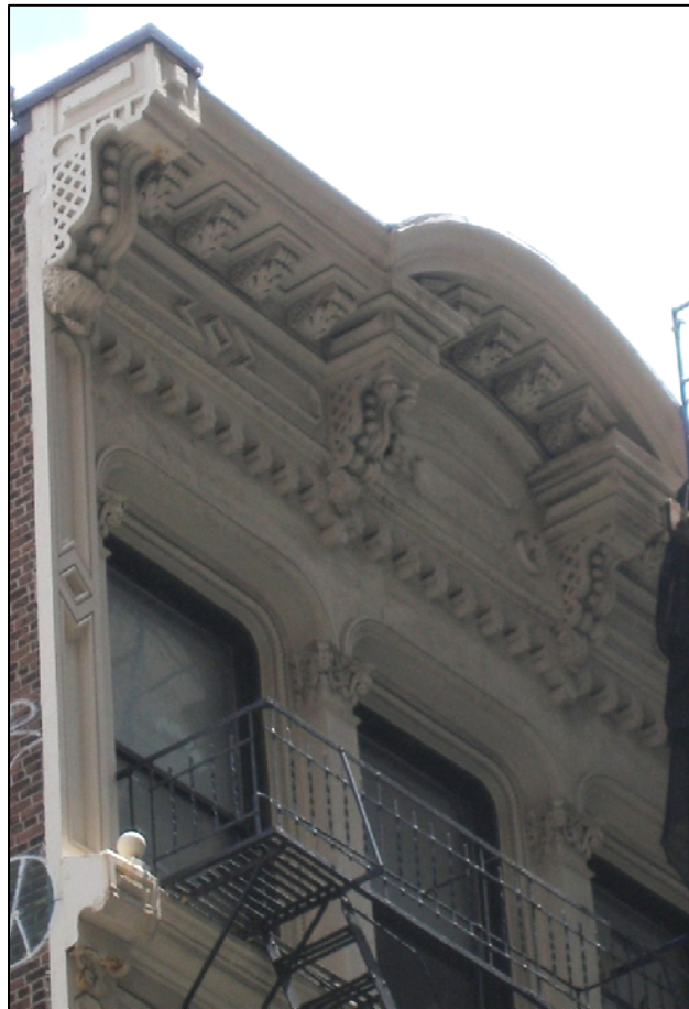
39 Worth Street Window and Cornice Details Photos: Christopher D. Brazee (top) and Marianne S. Percival (bottom), 2013
