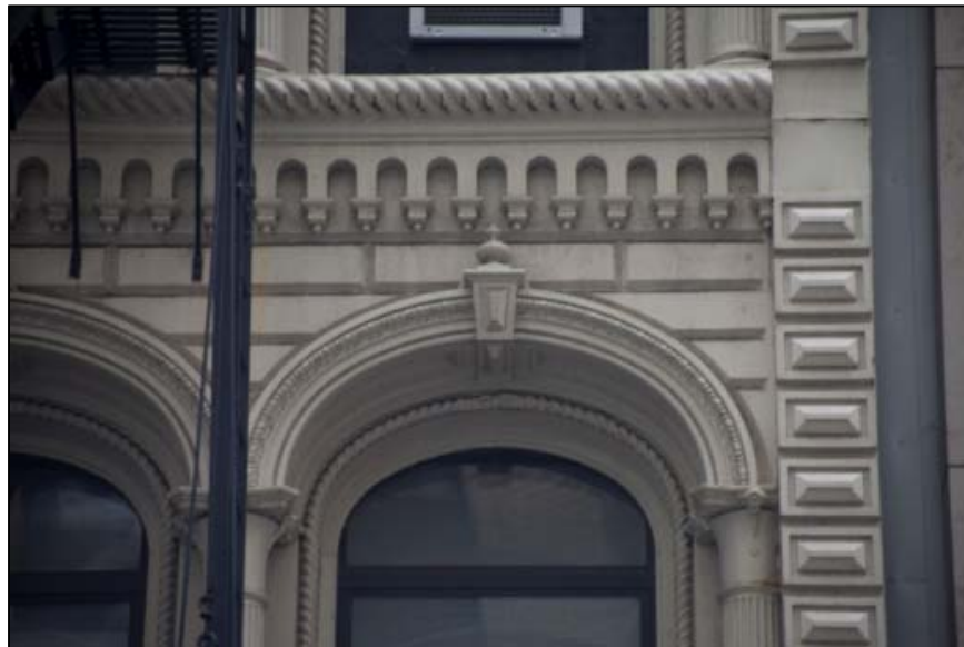
41 Worth Street Window, Facade, and Cornice Details Photos: Christopher D. Brazee, 2013
