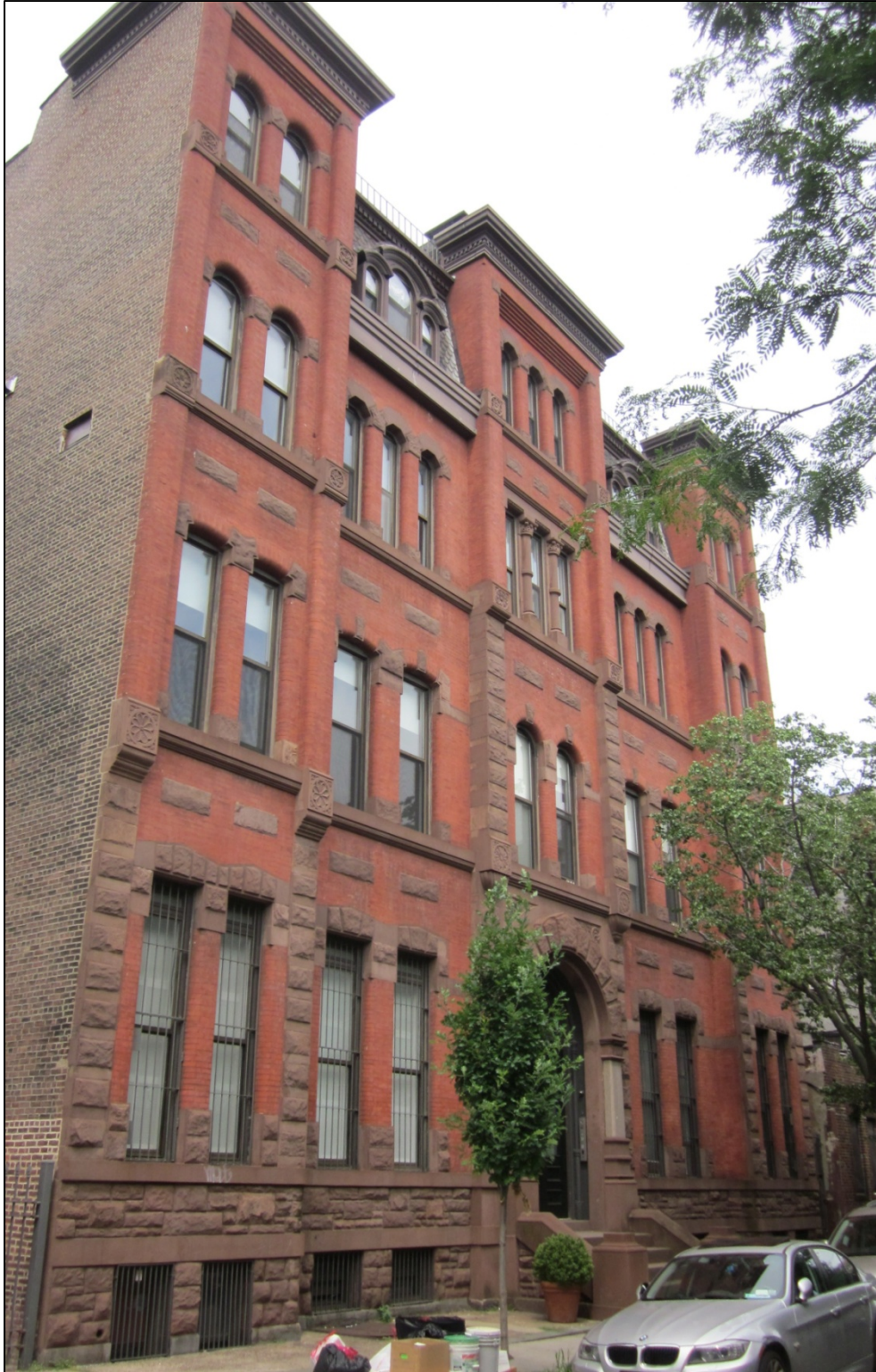
Long Island Business College 143 South 8th Street (aka 143-149 South 8th Street), Brooklyn Brooklyn Tax Map Block 2132, Lot 30 Photo: Michael Caratzas, 2013
