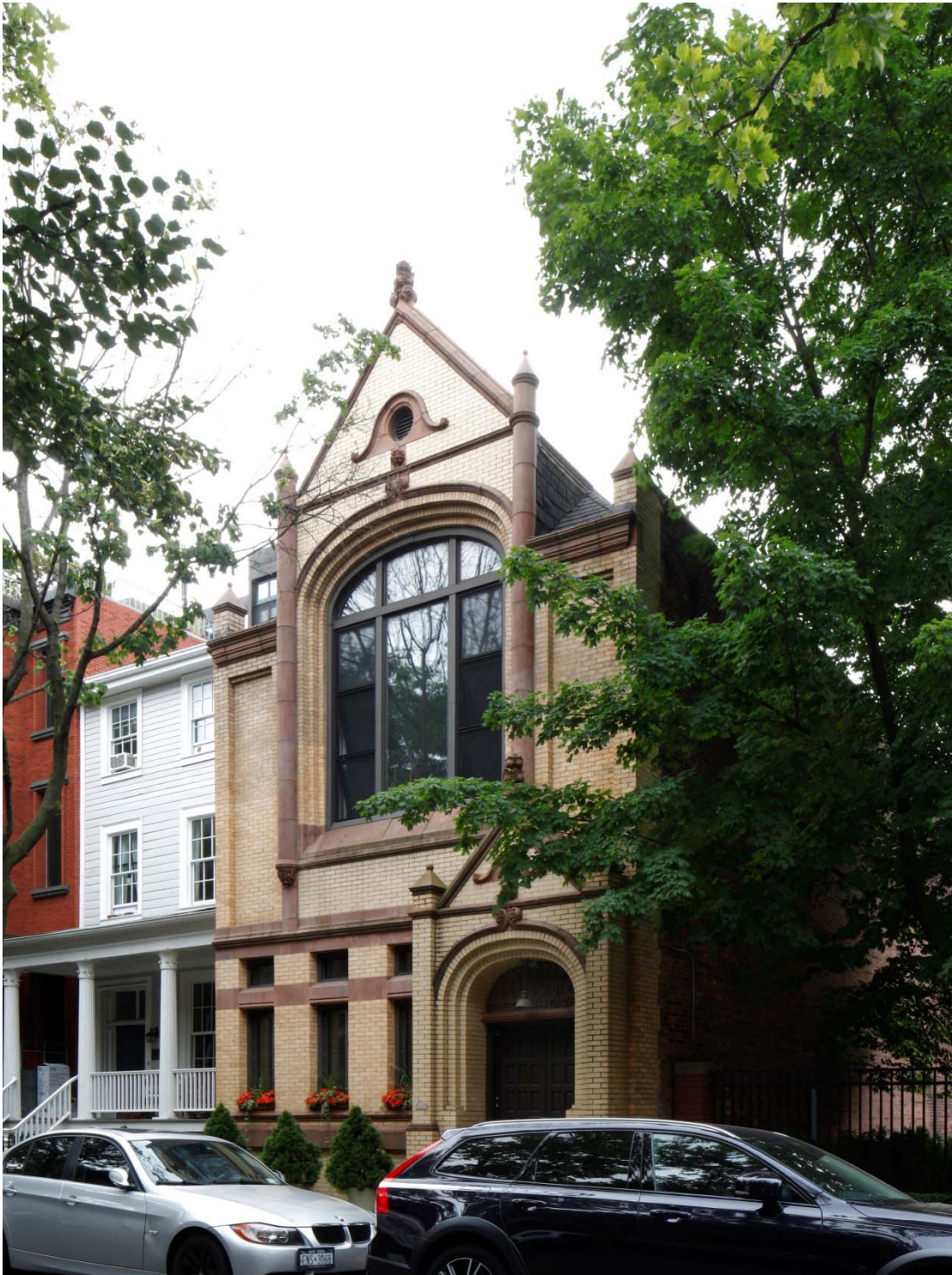
Figure 17, 358 Pacific Street LPC, February, 2017
