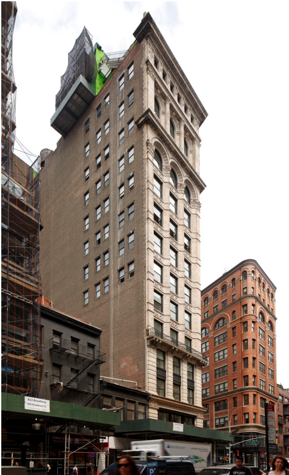
817 Broadway Building, South Facade, Sarah M. Moses, June 2019
