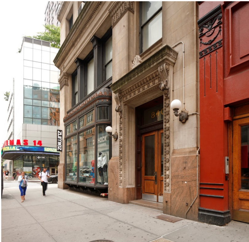
Base of 840 Broadway Building: East 13 th Street facade (above) and Broadway facade (below) Sarah Moses, June 2019
