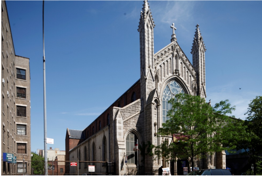
North and West Facades Fort Washington Avenue Jessica Baldwin, May 2021
