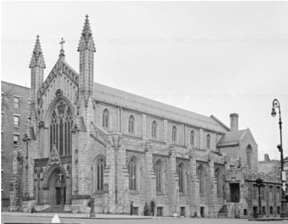
Holyrood Episcopal Church, c.1939-40 Tax Photograph, Municipal Archives, City of New York
