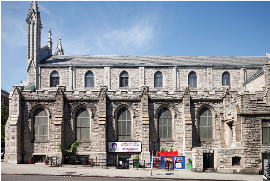
West 179th Street Facade (West End) Clerestory and Aisle Jessica Baldwin, May 2021
