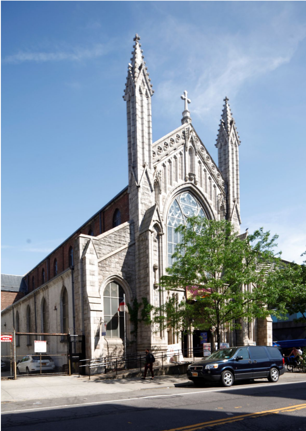
Holyhood Church – Iglesia Santa Cruz, 715 West 179th Street Fort Washington Avenue (West) and North facade Jessica Baldwin, May 2021
