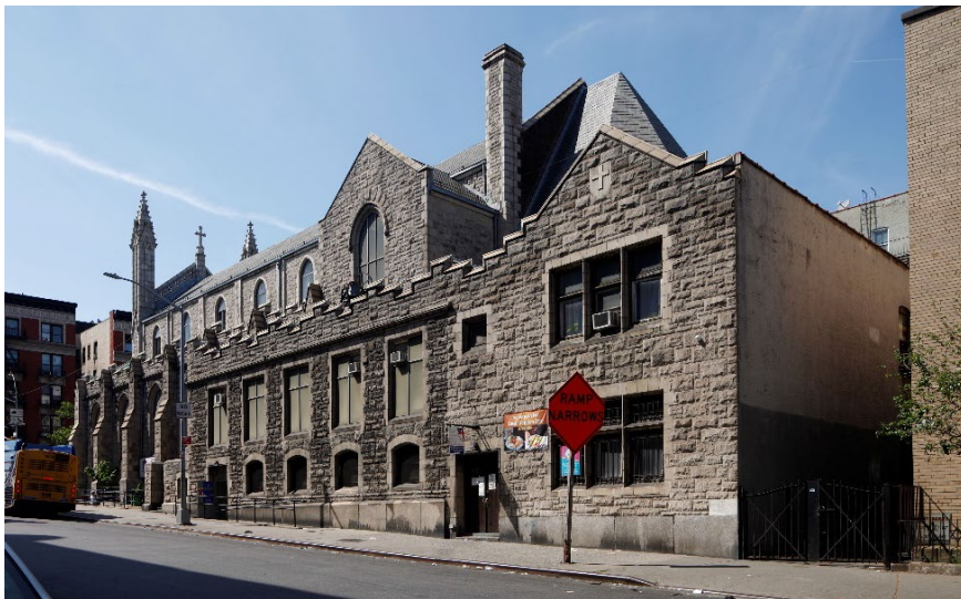
South and East Facades West 179th Street Parish House in Foreground Jessica Baldwin, May 2021
