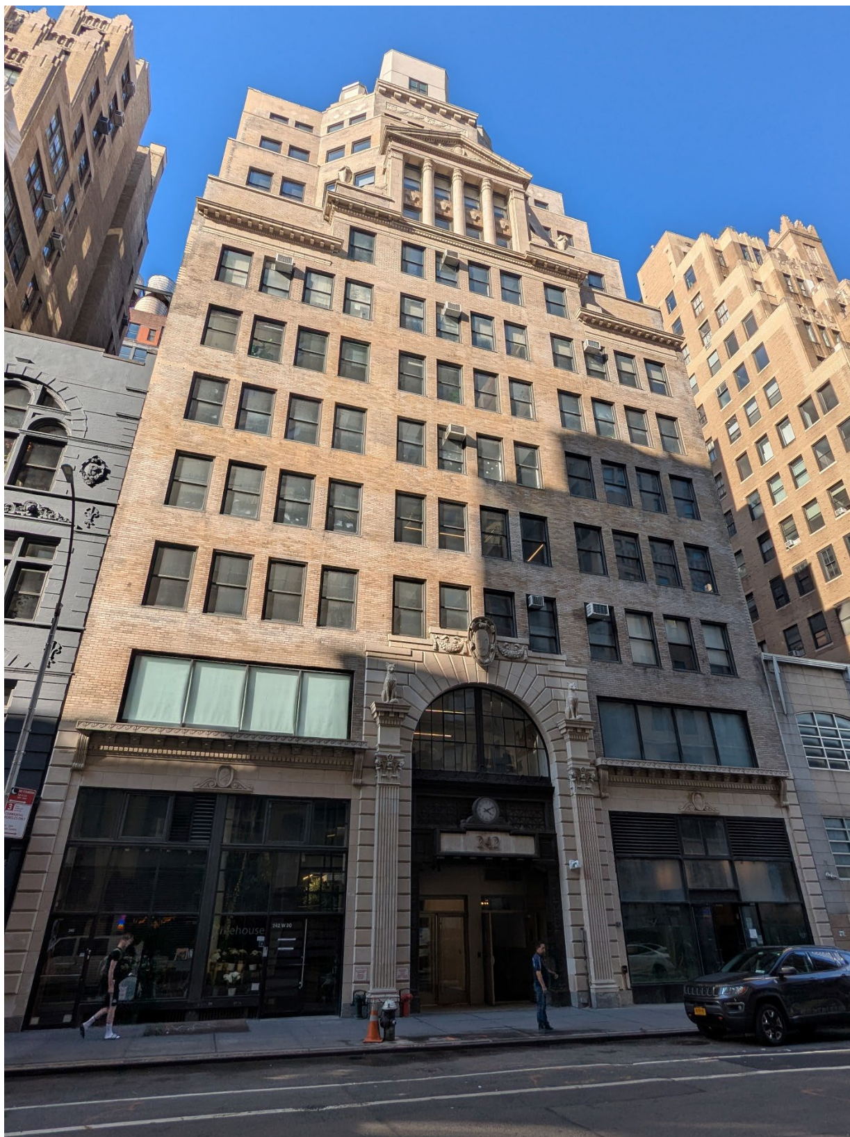
Furcraft Building, 242-246 West 30th Street, Manhattan LPC, August 2025
