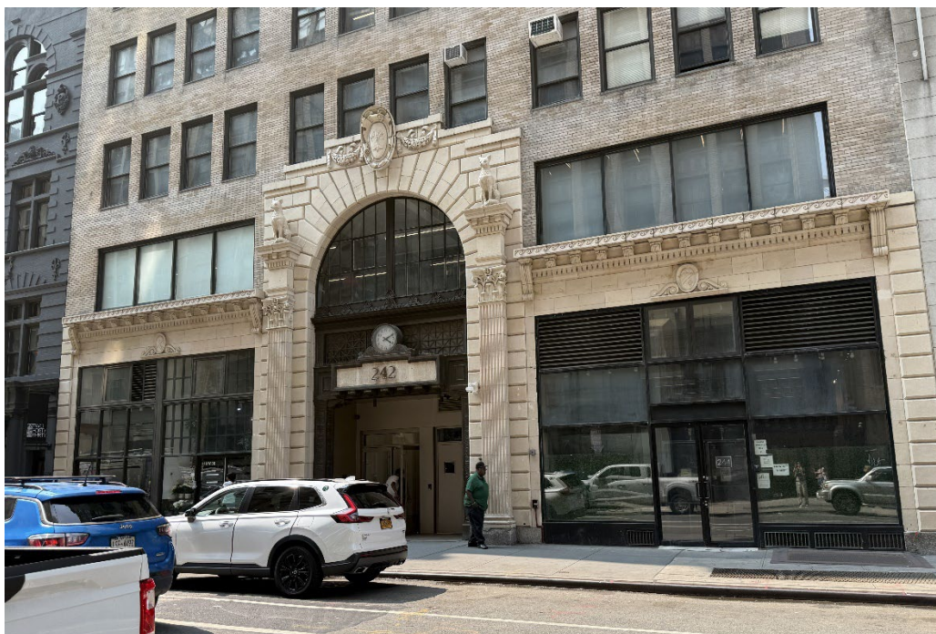
Base, including main entrance and storefronts LPC, August 2025
