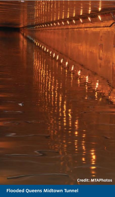
Flooded Queens Midtown Tunnel Credit: MTAPhotos (stillwater inundation, as opposed to destructive wave action), which tended to cause less structural damage and instead caused damage to building systems and contents. (See map: Location and Level of Building Damage )
