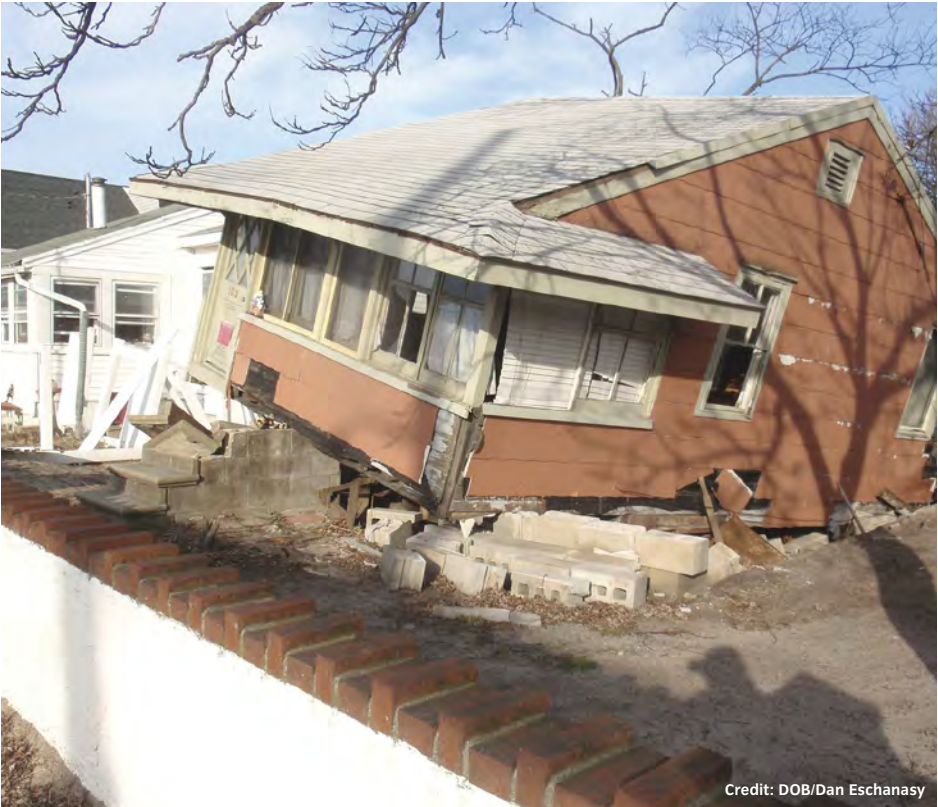
The effects of flooding and storm surge resulted in severe structural damage to many buildings during Sandy.
