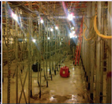
Cable vault of 104 Broad Street had to be stripped of copper wire post-Sandy.
