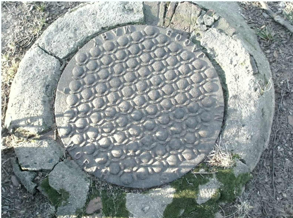
Photograph 15: Close up of manhole cover capping possible shaft feature from previous photograph. Note bricks under cement lining.
