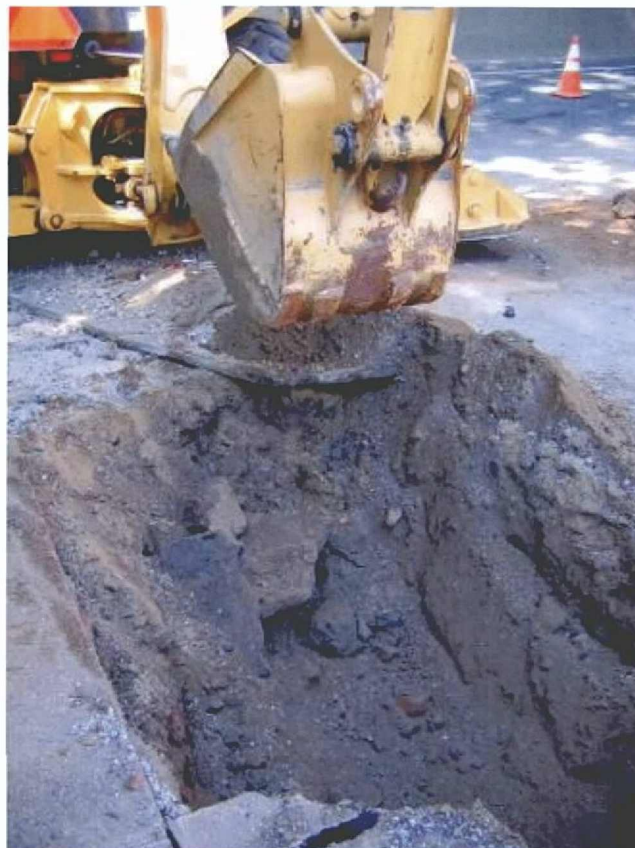
Photo 1 Start of sewer connection trench excavation south of the seawall with the connection visible at the top of the seawall (right) facing west.
