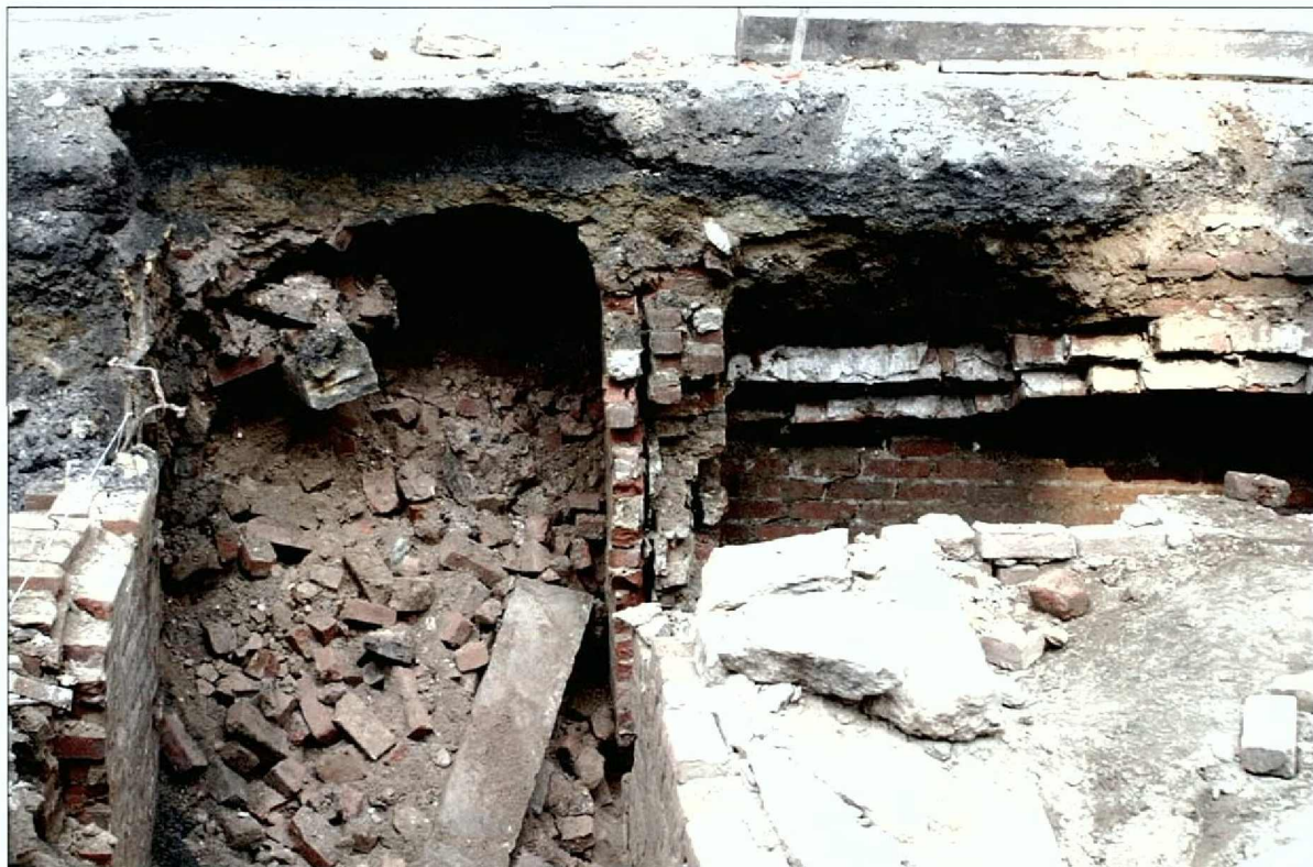
Looking west from the center of the areaway, towards the unexcavated rubble-filled void at the western end of the areaway. The vault, partially destroyed, is pictured on the right
