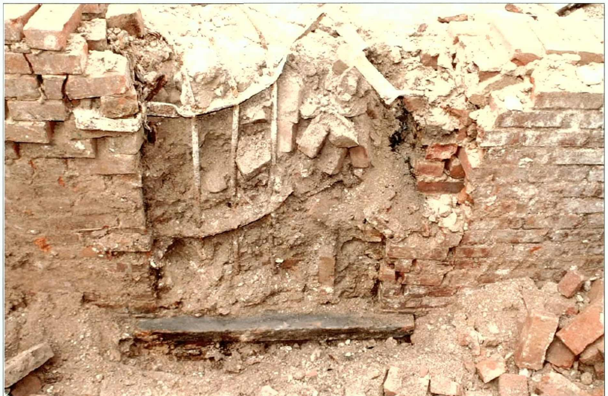
The central window on the (north) exterior basement wall of the former house that occupied the lot. The window has a stone ledge and iron bars. The upper portion of the window, located just below ground surface, was likely destroyed when the structure was demolished
