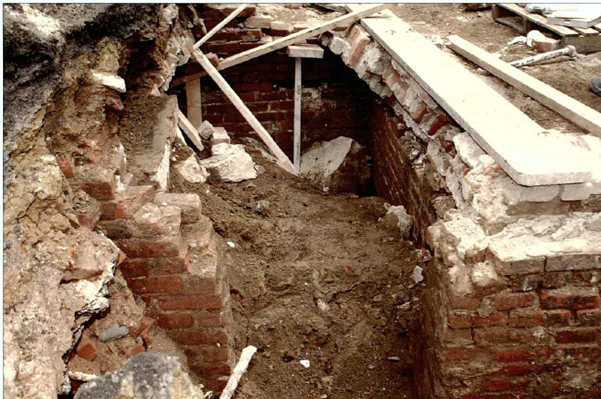
Looking north from within the western end of the area, through the vault entryway, into the vault. The north wall (center) and east wall (right) of the vault are visible, as is the partly destroyed ceiling of the vault. (Wood members pictured are part of a temporary shoring device)
