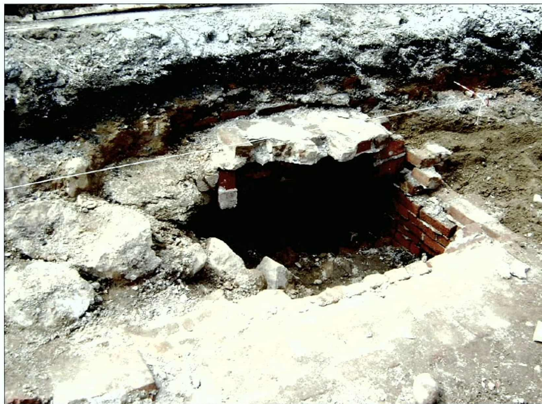
A view looking west towards the vault as it appeared on August 10, 2007, prior to the removal of its brick and stone roof, the large stones covering its southern half, and the rubble fill within it
