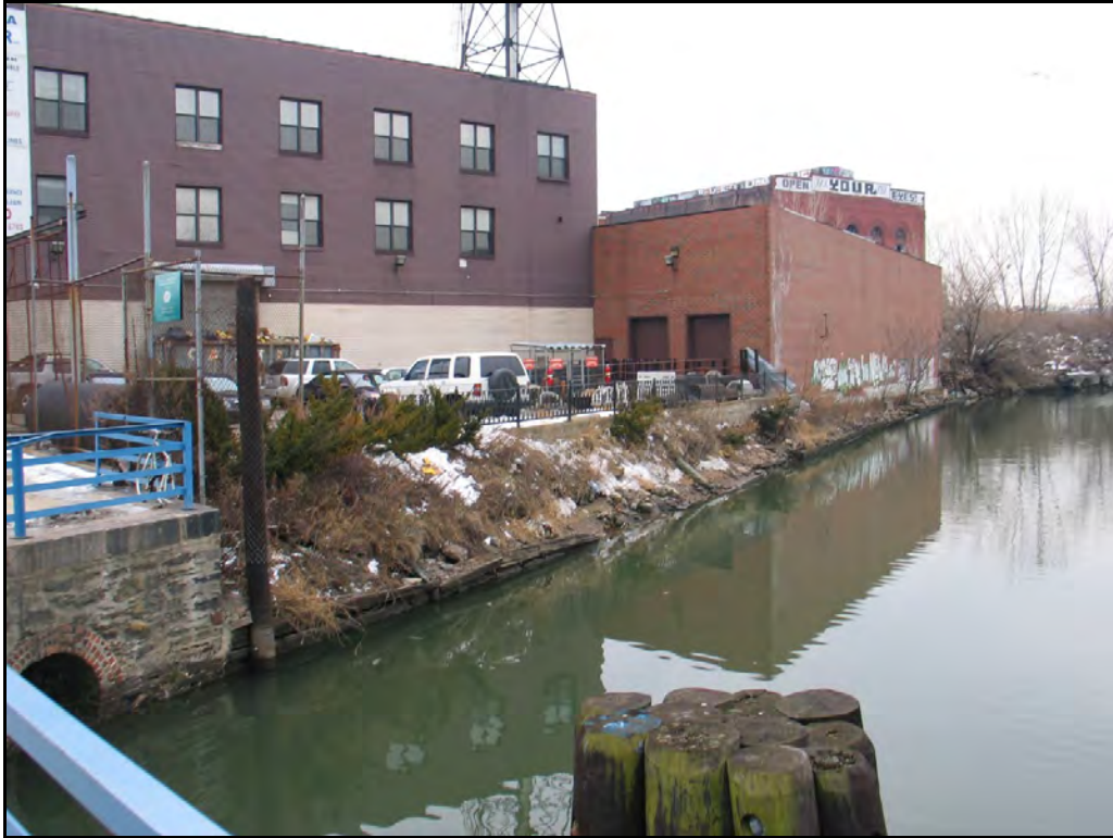
Photo 37: View of Gowanus Canal Bulkhead, Showing Deteriorating Upper Elements. View Southeast from Carroll Street Bridge.
