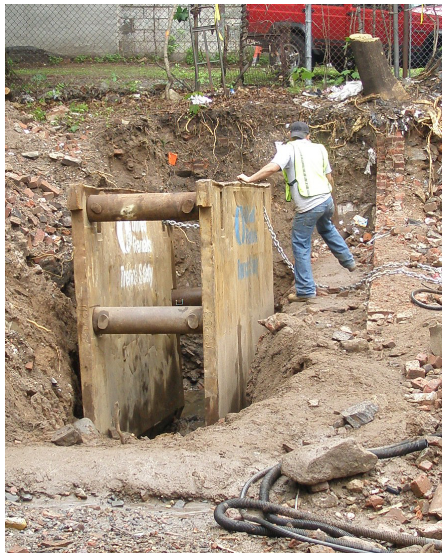
Safety walls placed in Trench 1 for hand excavation, looking west.
