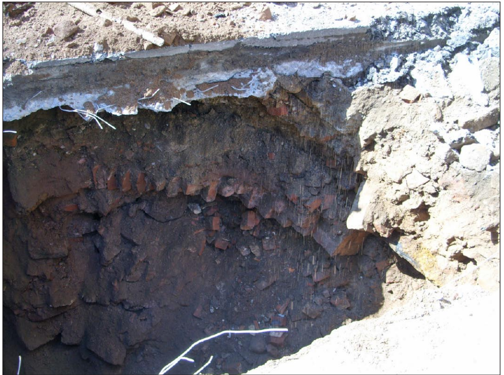
The brick arch of the vault shown in Photo 3, looking south from the approximate center of Gold Street, south of Ann Street
