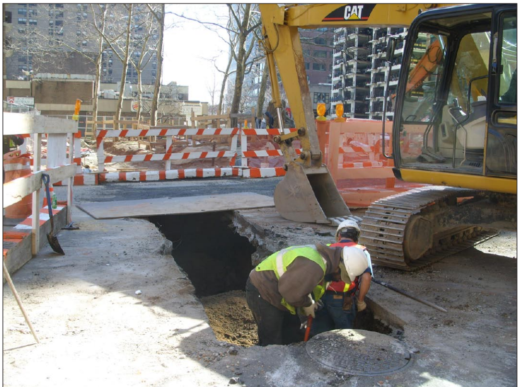
From the west side of Gold Street just south of Ann Street, a view looking west across Gold Street towards DeLury Square. The trench for drainage conduit installation is being excavated across Gold Street to connect with the existing sewer vault (sewer manhole shown in foreground)
