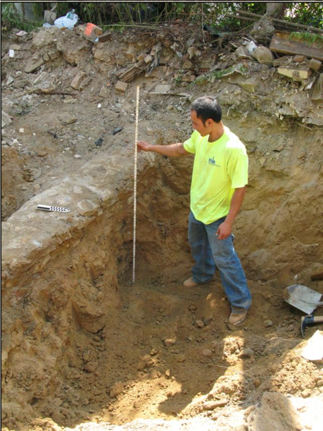
Fig. 29. The west end of TE-TT2, the stone foundation of the building formerly standing on the lot at the end of excavation
