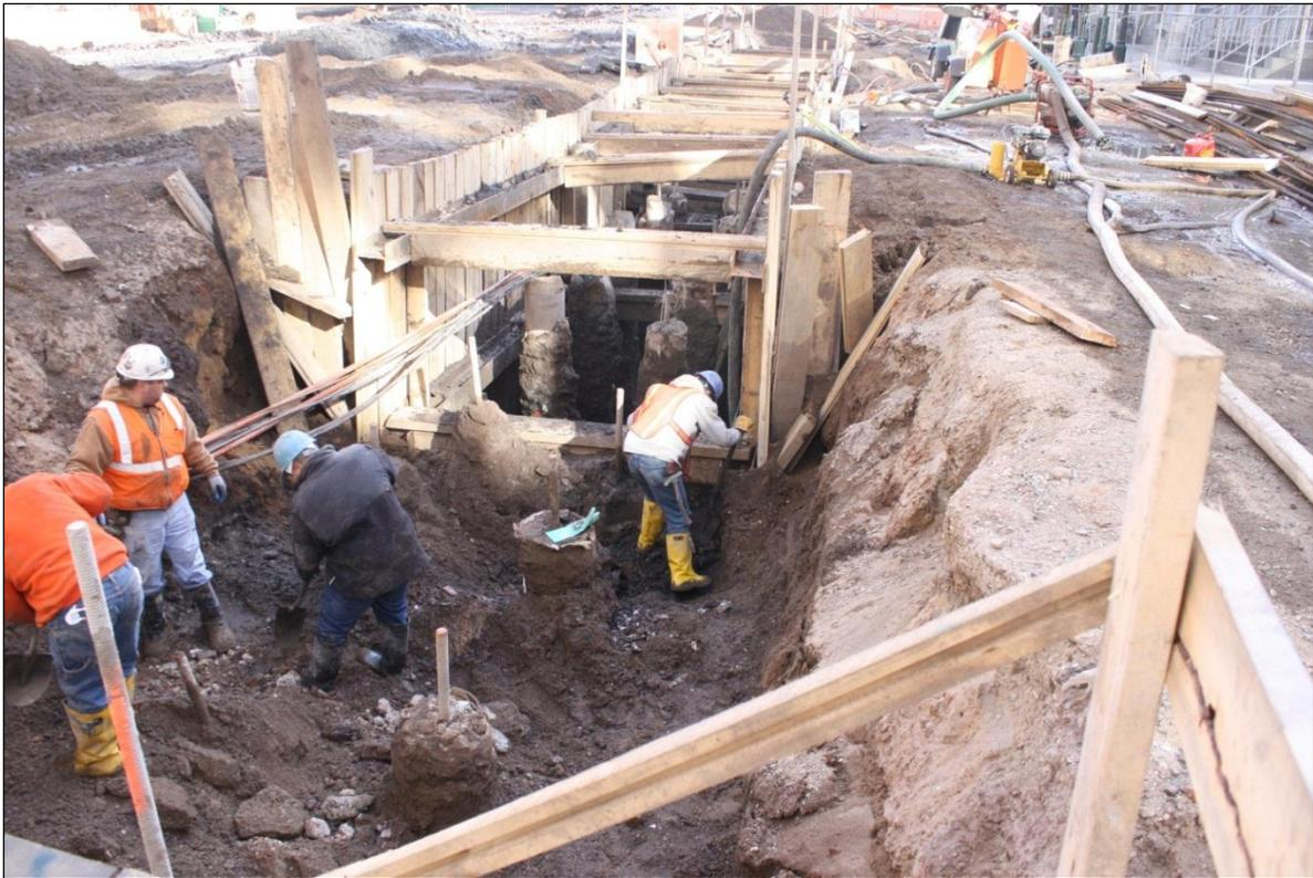
Image 24: Excavation Unit 7 – showing area of wall collapse
