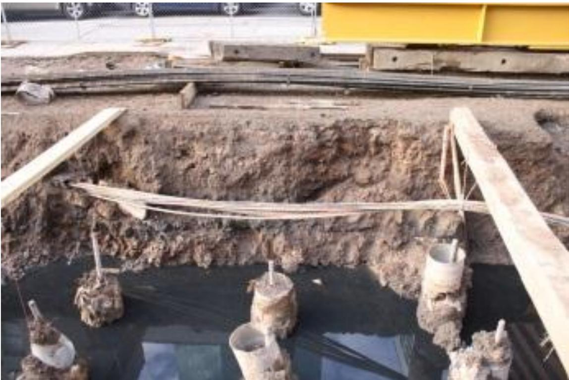
Image 32: Both utility lines and water intrusion in the trench
