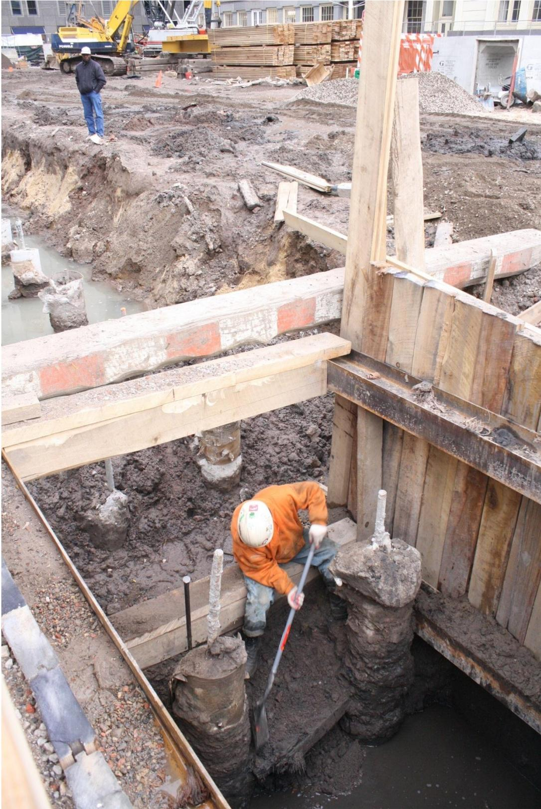
Image 54: clearing away the concrete column support
