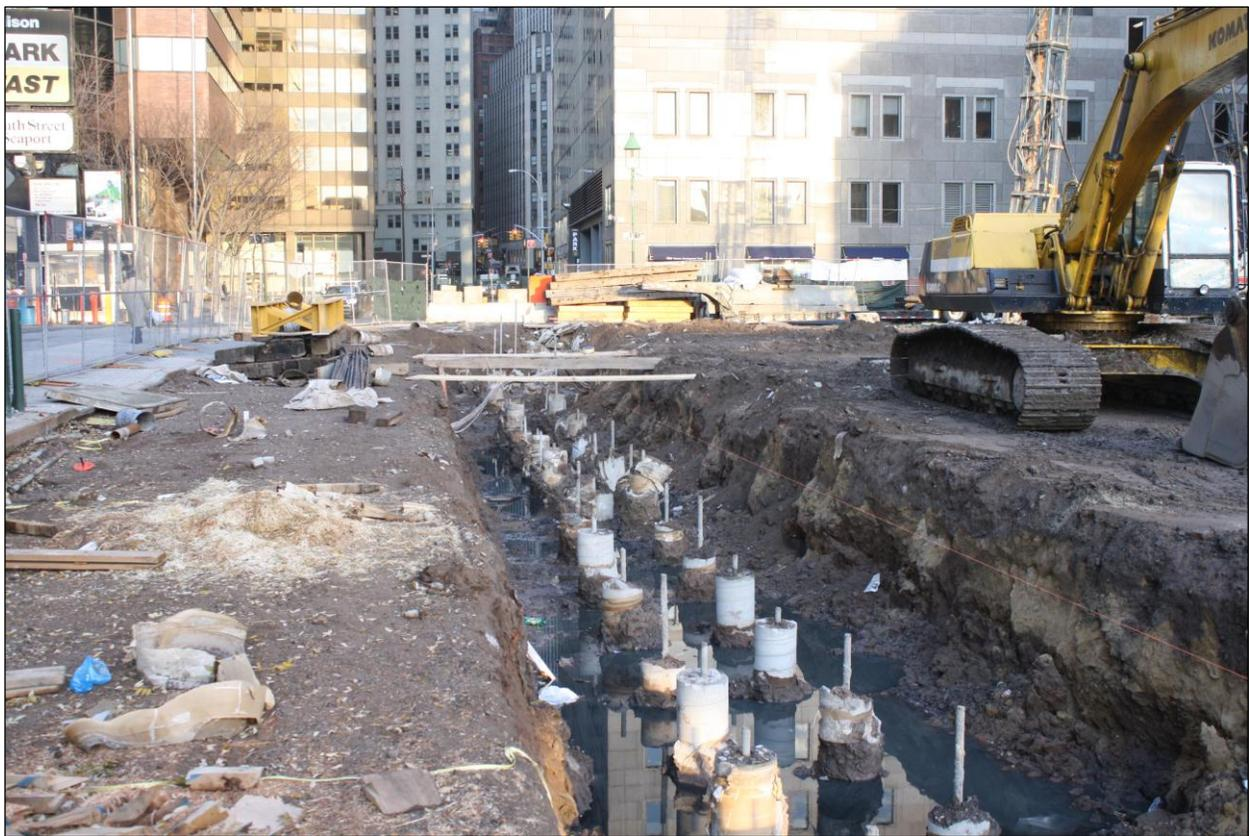
Image 02: John Street, looking west during pile driving operation – note the ground water intrusion
