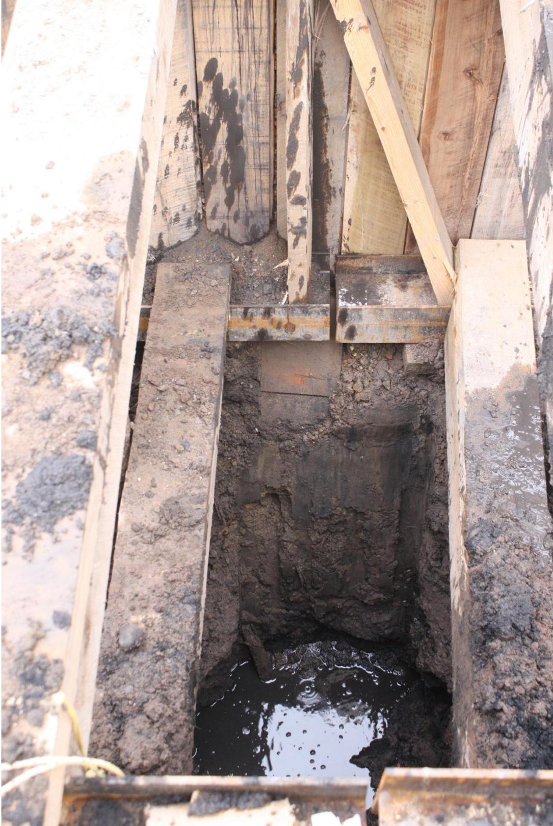
Image 52: muck and mud at the bottom of the trench
