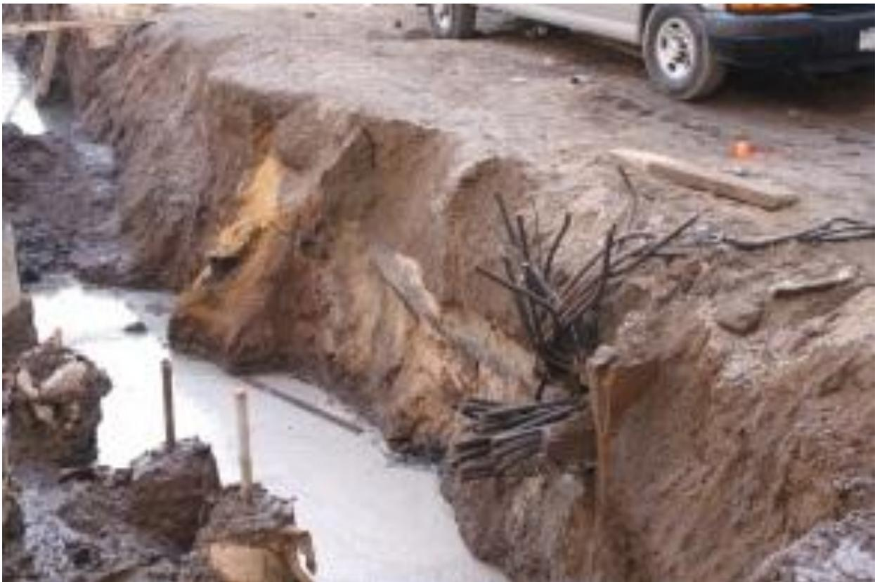
Image 29: Ground water intrusion, coupled with previous utilities were a constant throughout the site
