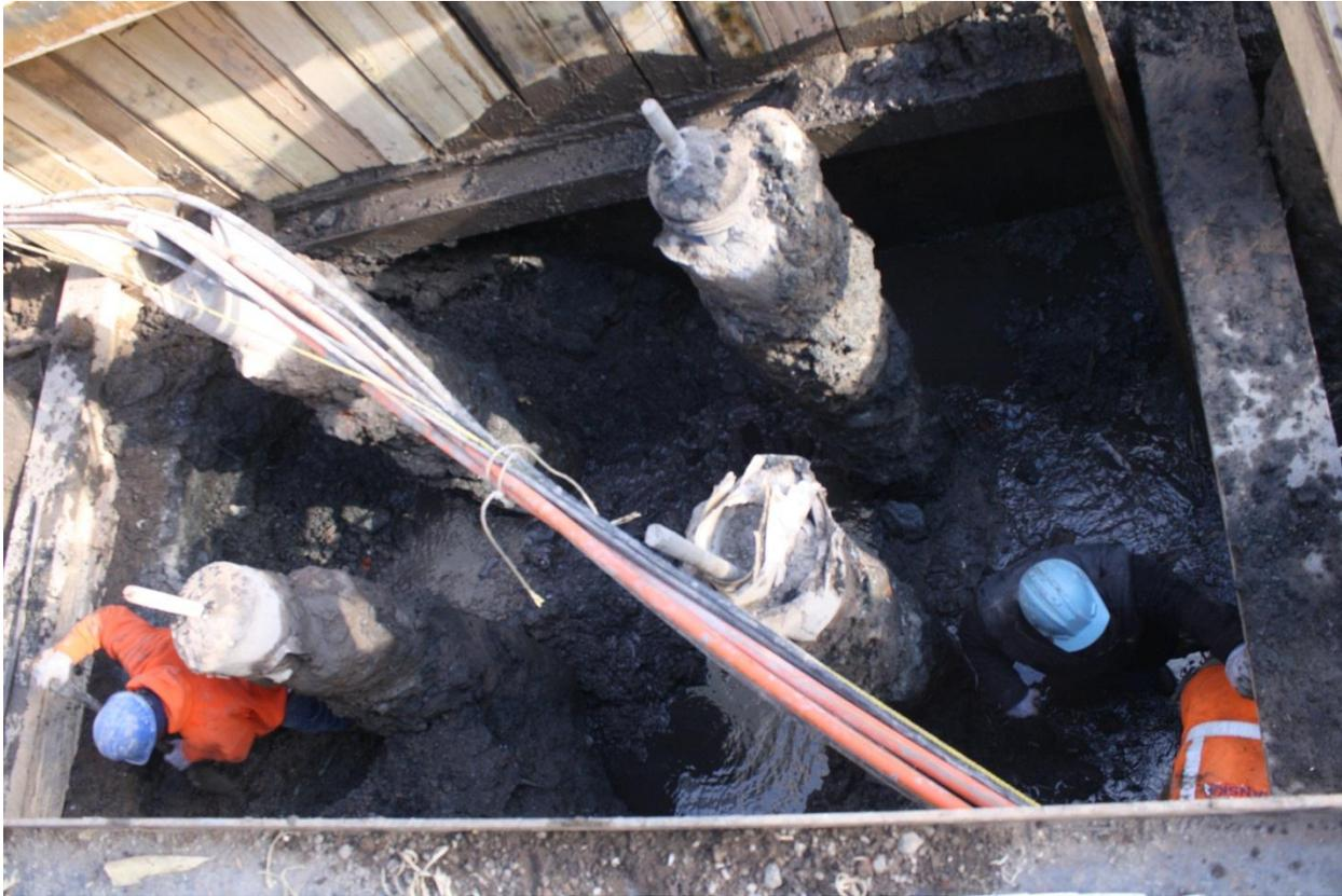
Image 06: Soil conditions during active de-watering
