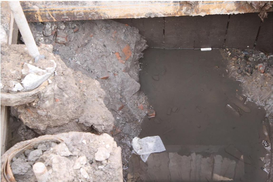
Image 46: general example of ground water intrusion
