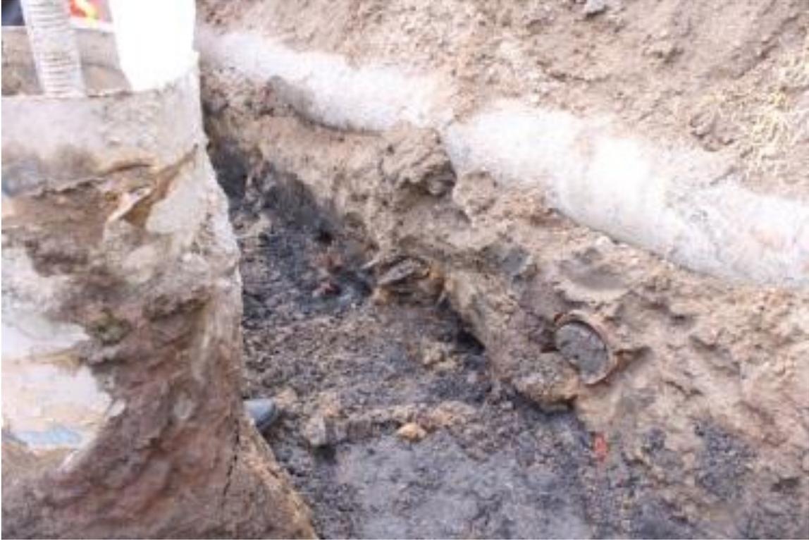
Image 31: note the existing water line intrusion and brown silted water
