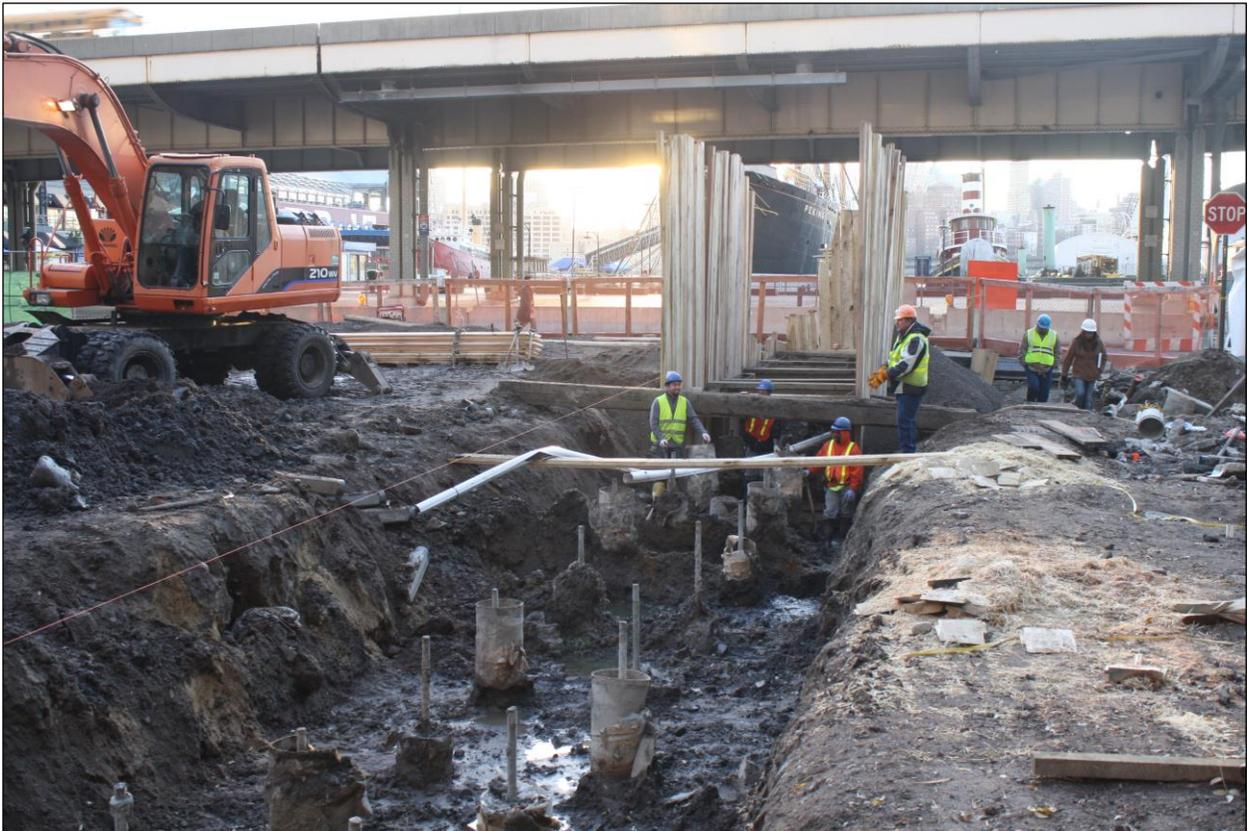
Image 03: John Street trench, looking east, showing concrete piles and twenty-foot (20') sheeting boards prior to being driven into the ground for trench shoring.
