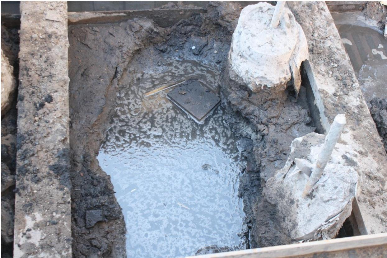
Image 04: Water continually filled the excavation trench
