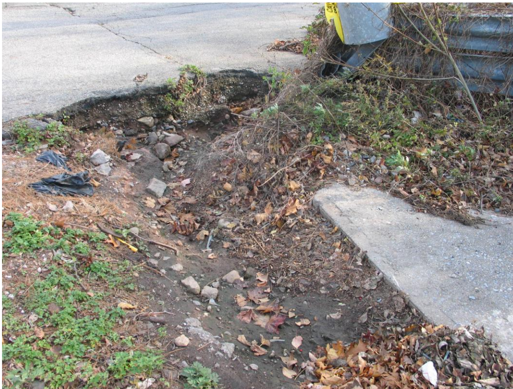
Photograph 4: Evidence of erosion at edge of Amboy Road cul-de-sac where concrete culvert begins. View looking southwest.
