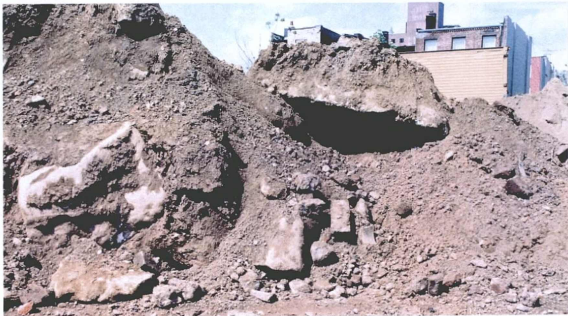
Photo 6: Large pieces of concrete and asphalt excavated from eastern end of Trench B.
