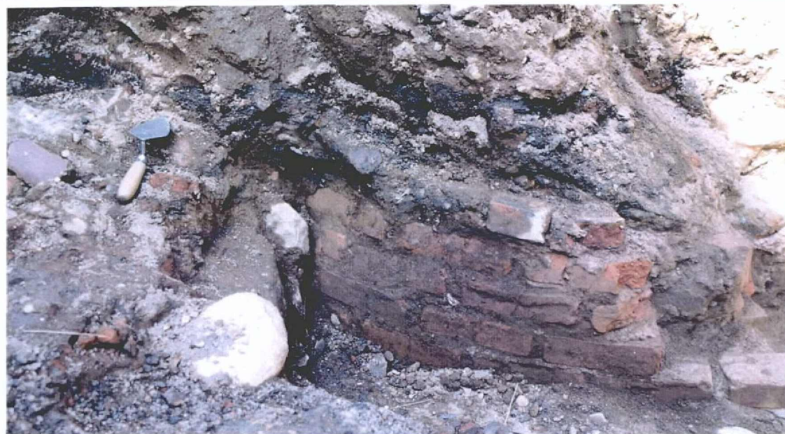
Photo 8: Brick cistern located immediately east of brick and stone foundation wall seen in Photo 7.
