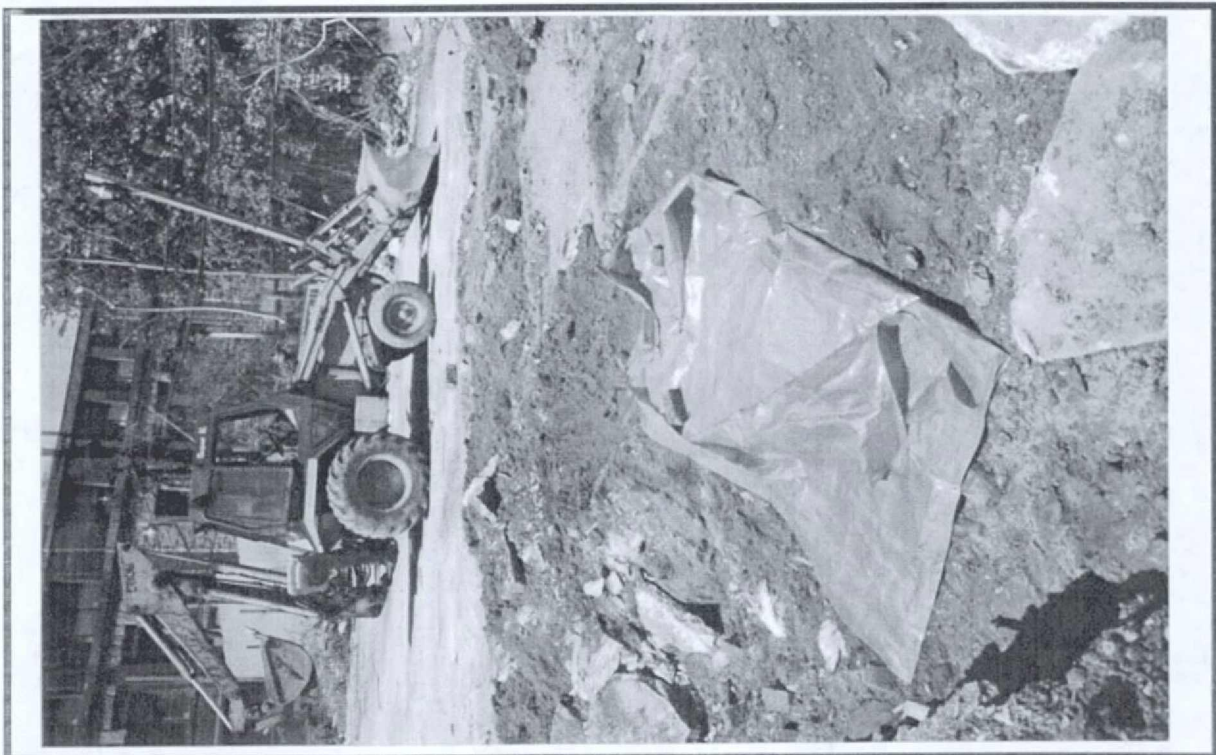
Photo 10: Cistern was covered with tarp and protective layer of soil placed over it.
