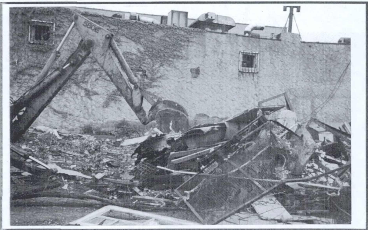
Photo 2: Debris was piled on front of lot in area of former house for later removal. Soil that had been dumped on property was carefully removed to expose original land surface.
