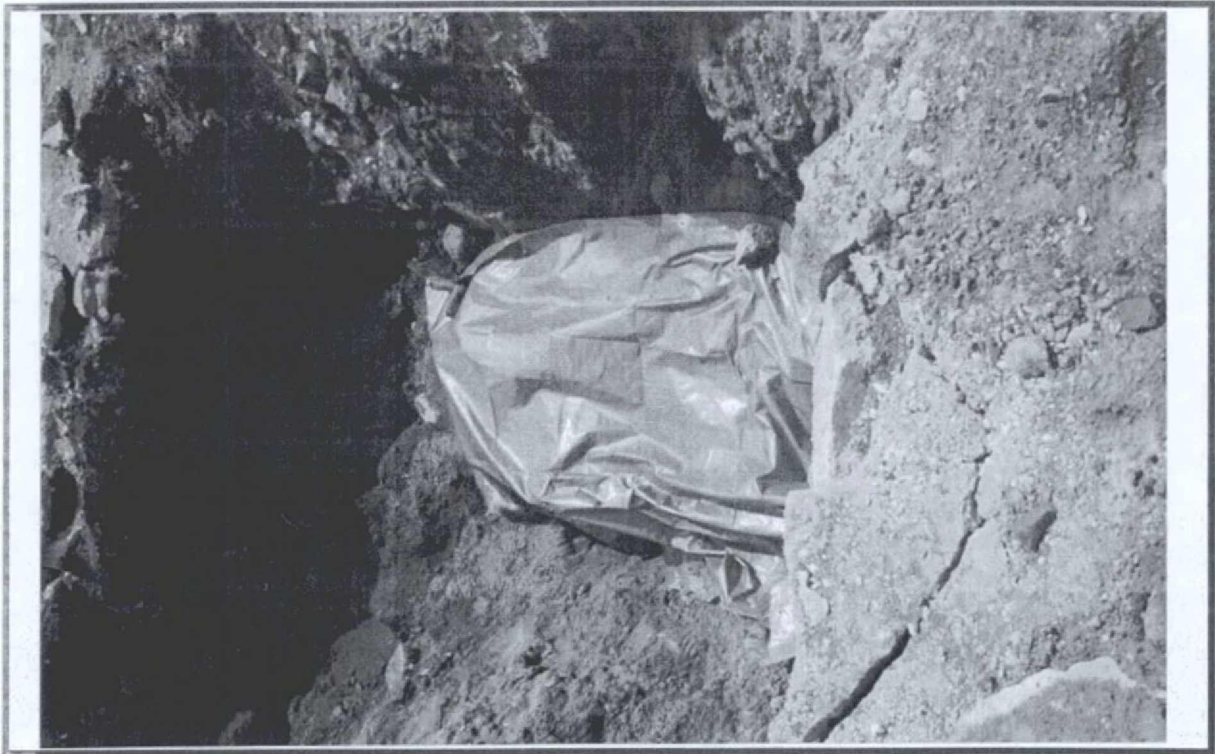
Photo 15: To facilitate further investigation, if it was deemed warranted, the stone foundation was covered with a tarp and a protective layer of soil placed over it.
