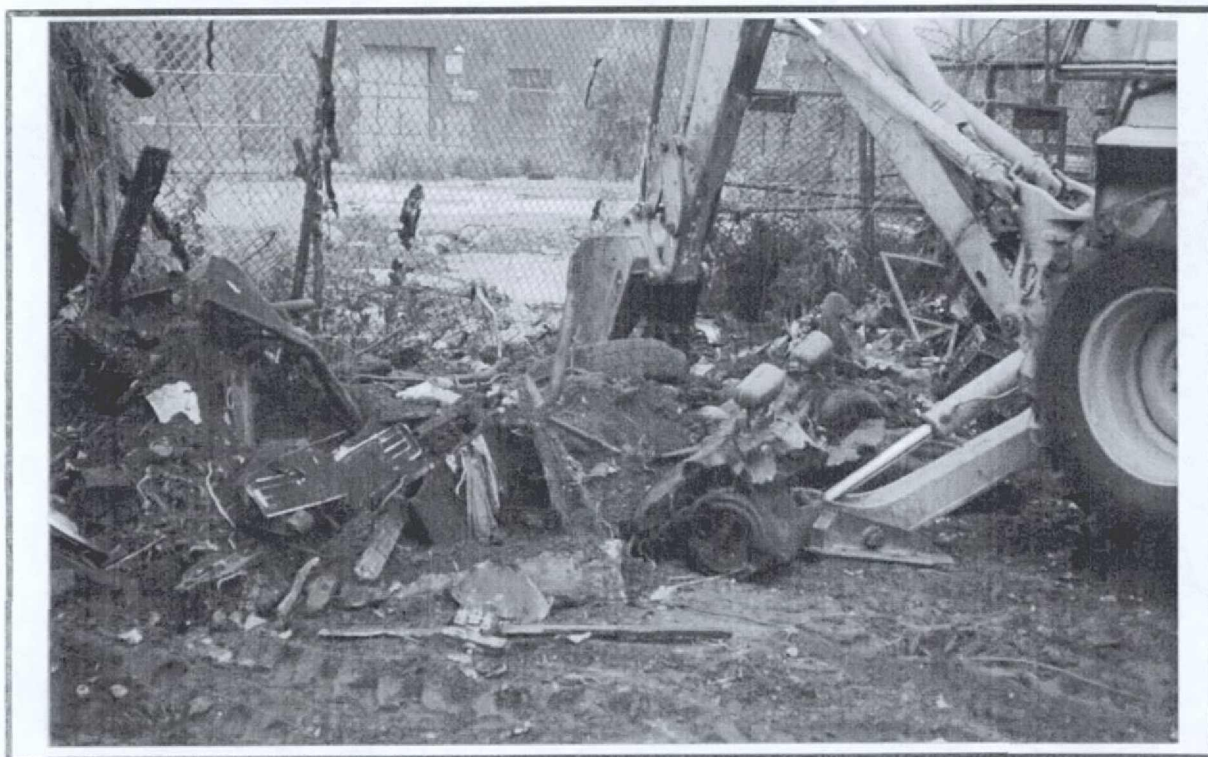
Photo 24: At rear of lot extensive debris been bulldozed against the property line fence. The soil was filled with automobile parts, broken bedsprings, and the like. All of this had to be removed to expose the historic ground surface for excavation.
